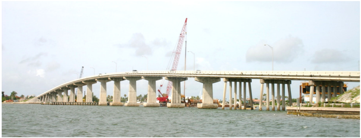
Figure 2. Pile cap and column- and pile bent-type piers (built 1969).
