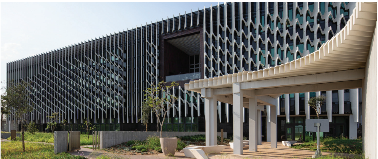
The new U.S. embassy in Maputo, Mozambique, uses precast ultra-high-performance concrete to meet durability and blast resistance requirements. Courtesy of Pernix Federal LLC.
