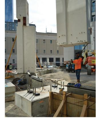
Coordination, fabrication, and placement of the Fred D. Thompson U.S. Courthouse and Federal Building rotunda precast concrete columns was one of the key design challenges. Courtesy of GATE Precast.
