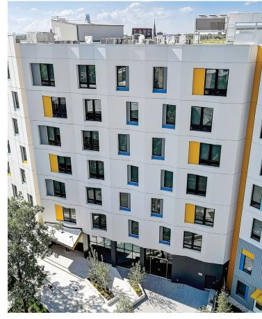
With limited access to this urban site, totally prefabricating the components of the Lucy Gonzalez Parsons Apartments, a seven-story multifamily residential complex in Chicago, Ill., ensured quality control and facilitated construction scheduling. Courtesy of Wells.
