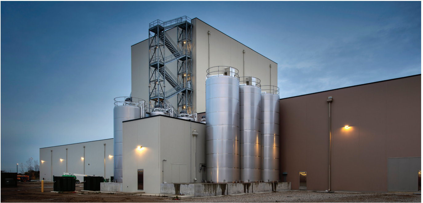
The MWC LLC processing facility dryer structure is constructed of precast concrete. Courtesy of Shambaugh & Son LP.
