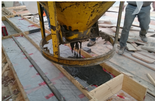
Placing the UHPC
