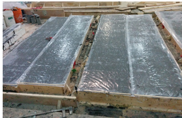
Freshly placed concrete covered with plastic
