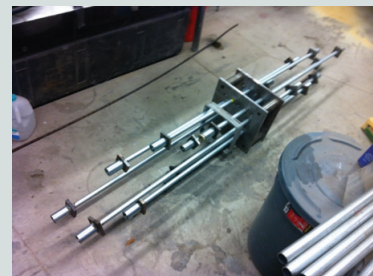
Figure 9. Splice header with staggered ducts and embedded chuck assemblies. All post-tensioning ducts are the same length.
