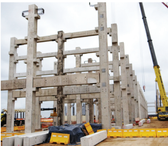
Figure 14. Erection of the precast concrete columns and beams.
