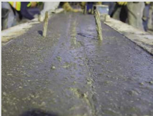
Beam surface consistency immediately after casting
