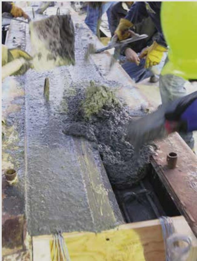
UHPC consolidation around reinforcement
