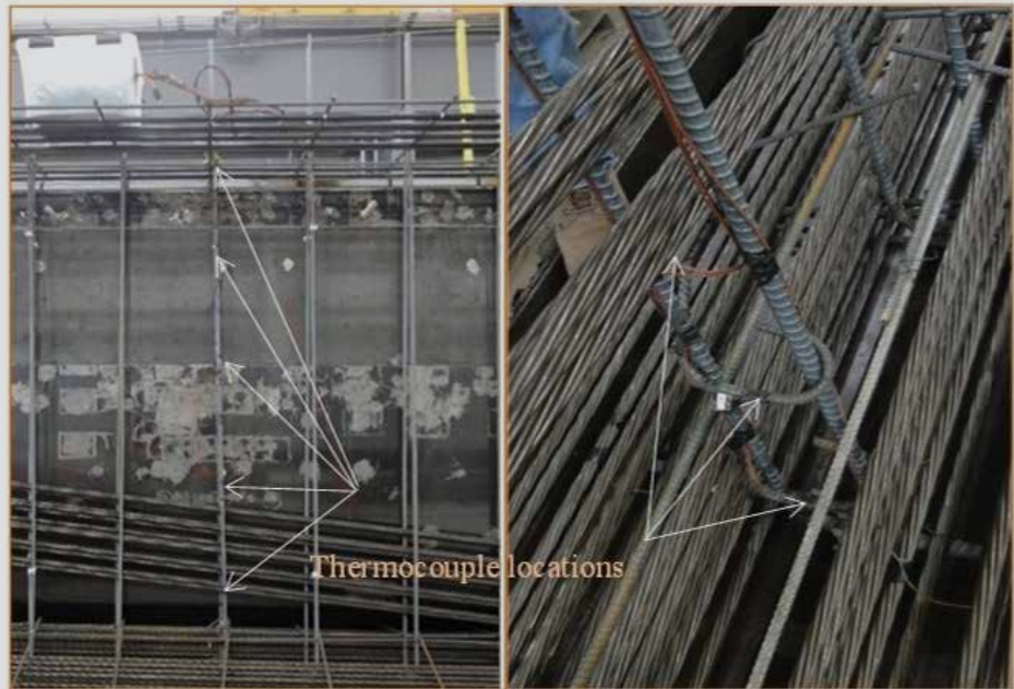
Figure 2. Thermocouple locations. Note: B = bottom of girder; C = center of girder; L = left side of girder; LW = lower web; R = right side of girder; T = top of girder; UW = upper web.
