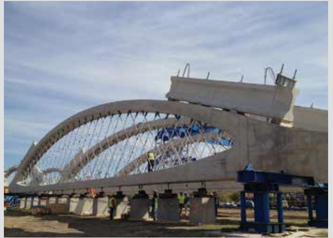
Arrangement of hydraulic rams and strongbacks during upward jacking
