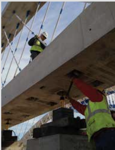
Retightening the hanger nuts when the rams were activated
