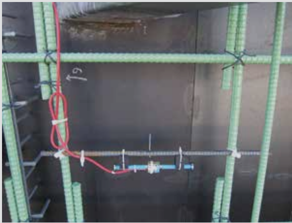
A vibrating-wire gauge tied to the arch reinforcement
