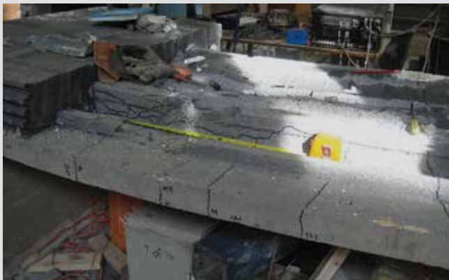
Crushed web in BPS
