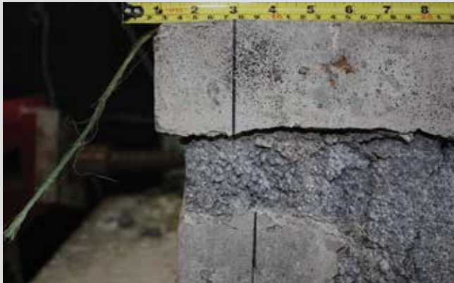
Visible slip after failure of BPF
