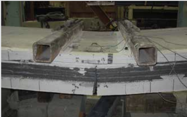
HPF after rupture of structural wythe reinforcement
