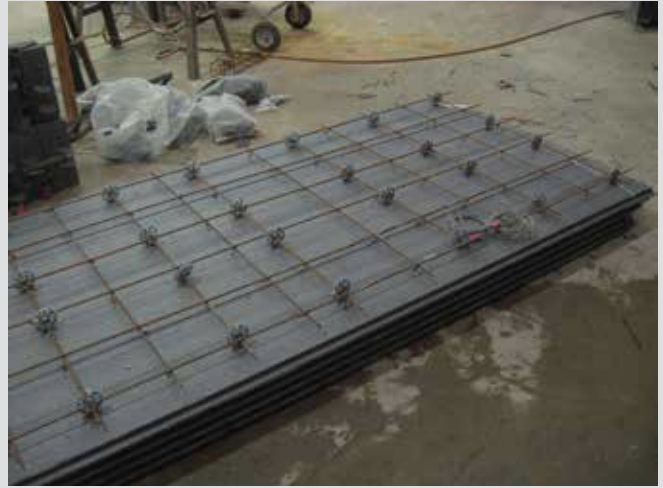
Foam and facade reinforcement
