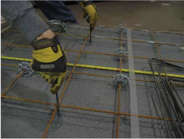
Inserting basalt-fiber-reinforced polymer shear connector
