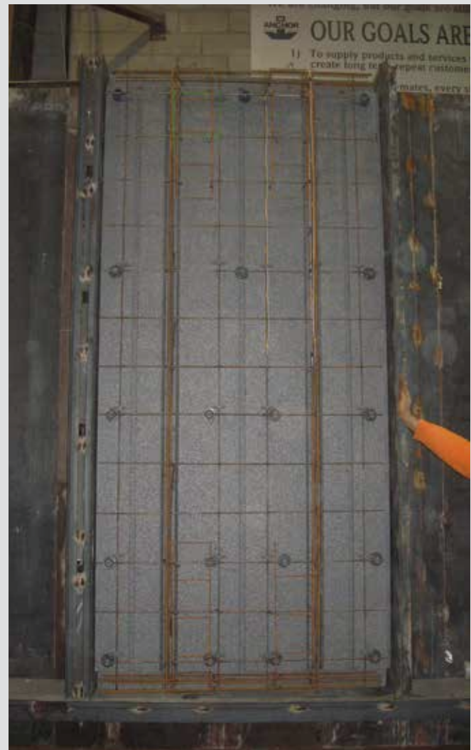
Foam and reinforcement before closing of form
