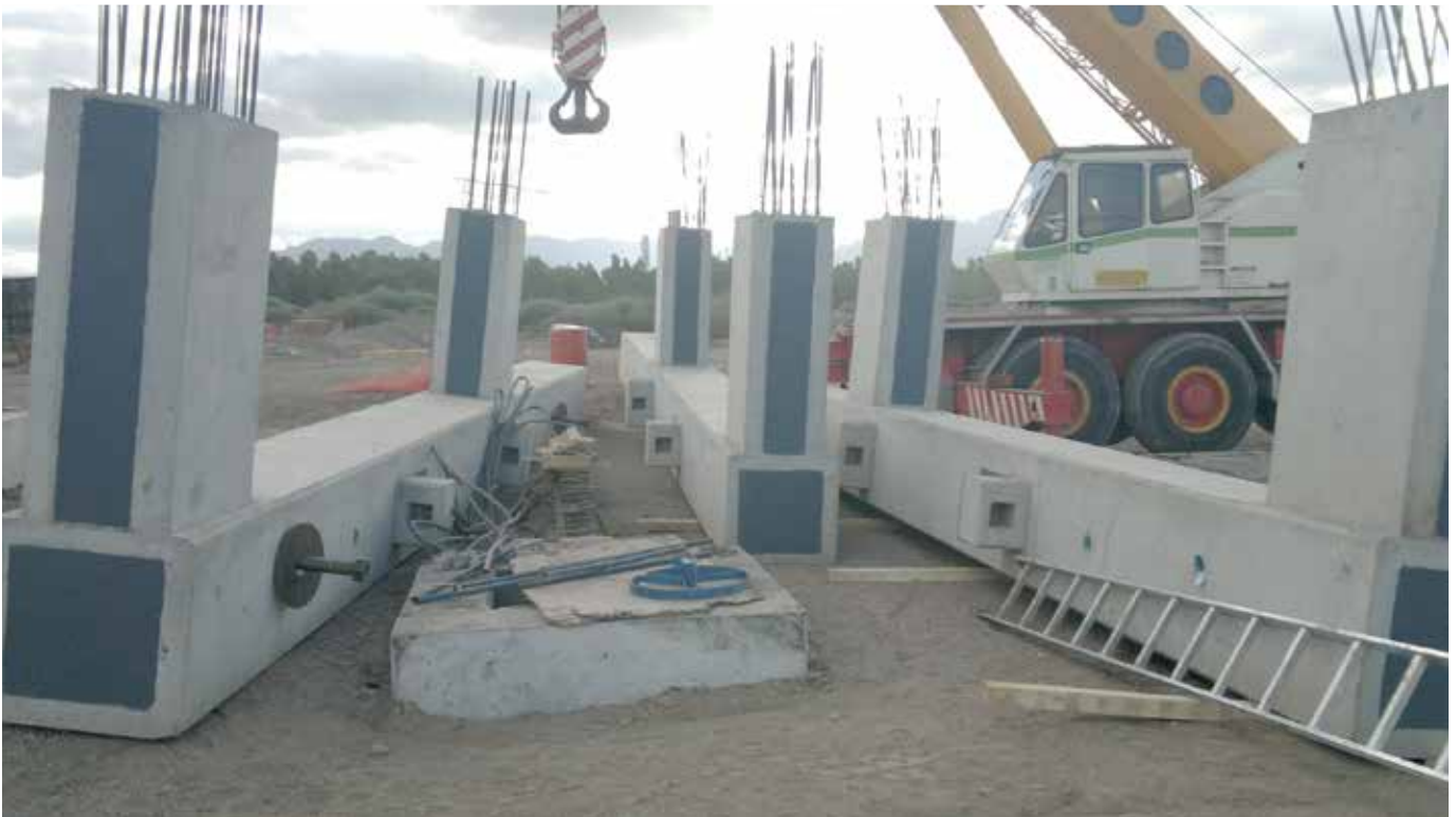
Figure 11. F-shaped precast concrete elements.
