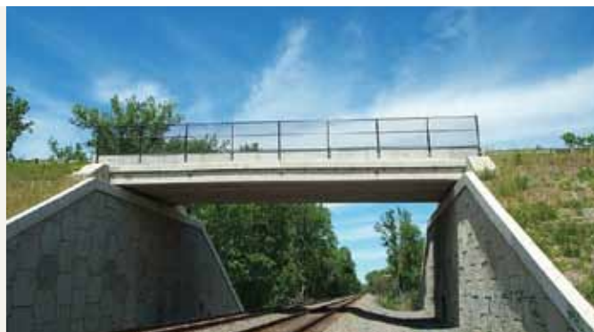
Figure 1. A single-span box-beam bridge was used for Schodack Island Road over Conrail tracks in New York state. Photo courtesy of the New York State Department of Transportation.
