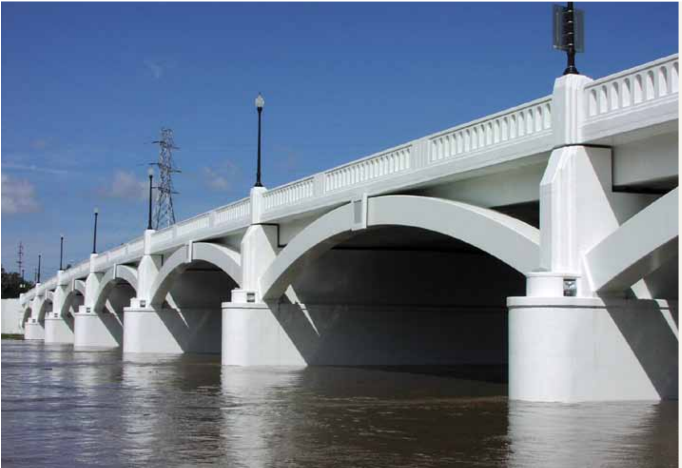
Figure 3. An adjacent box-beam bridge with facade arches was used to replicate an arch bridge in Ohio.
