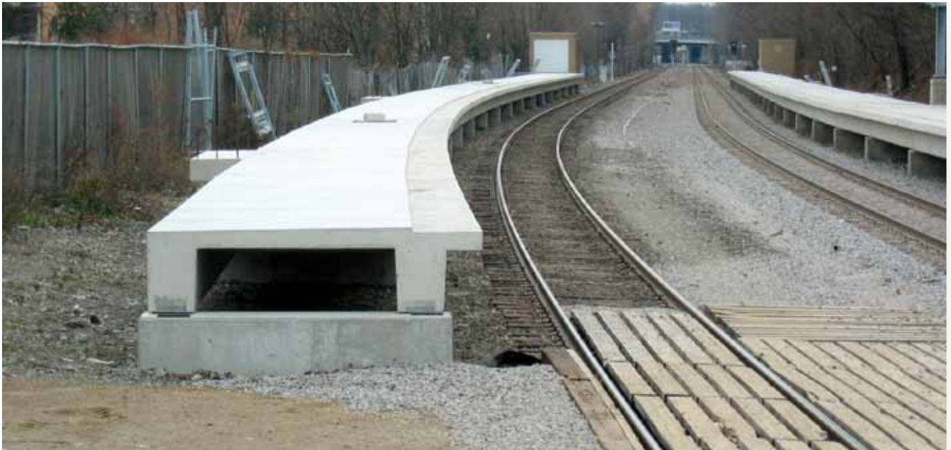
Figure 1. A high-level railroad platform slab inspired the model for the northeast extreme tee beam.
