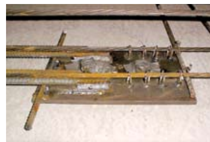
Fig. 11. Back of the base embed plate.
