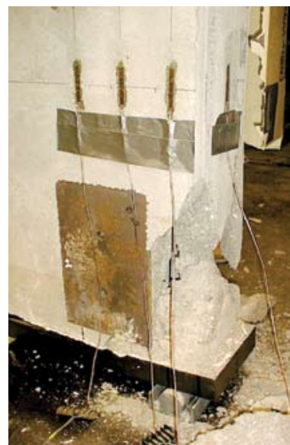
Fig. 17. Typical failure of compression test prism.
