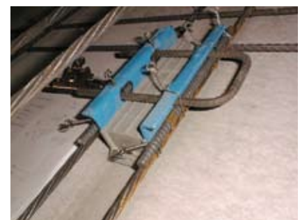
Fig. 7. Anchorage of slotted insert.
