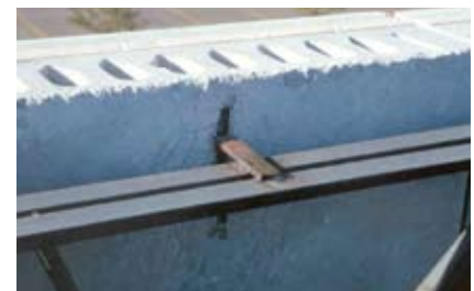
Fig. 6. Corewall attachment to roof.
