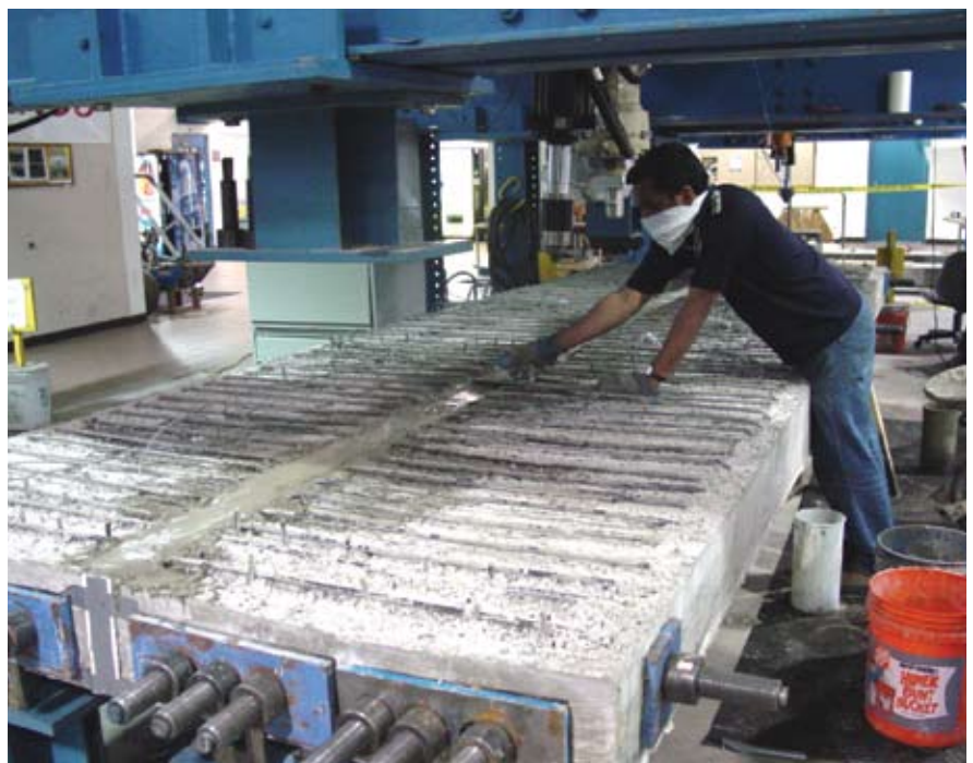
Fig. 6. Grouting of longitudinal joint between two box beams.
