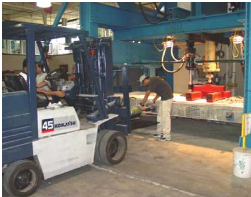
Fig. 9. Transverse post-tensioning of bridge model BBD-1 after casting of the concrete deck slab.
