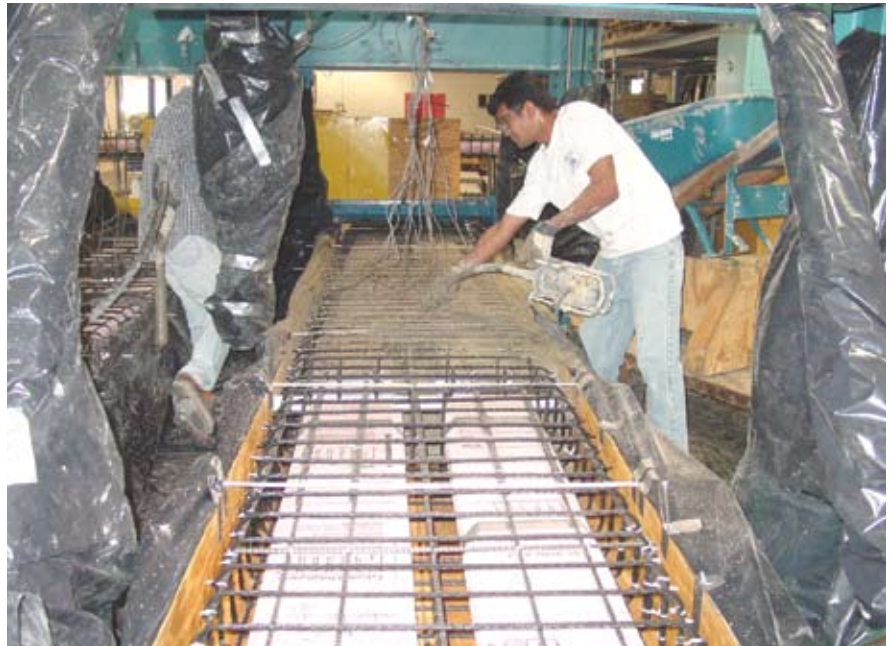
Fig. 5. Placement of concrete in the formwork after pretensioning of tendons.
