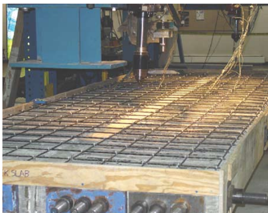
Fig. 8. Bridge model BBD-I before the concrete deck slab casting.
