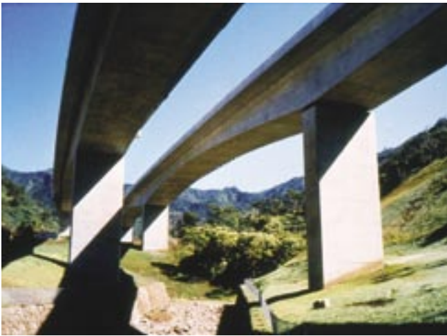
Fig. 16. North Halawa Valley Viaduct (from Reference 7).
