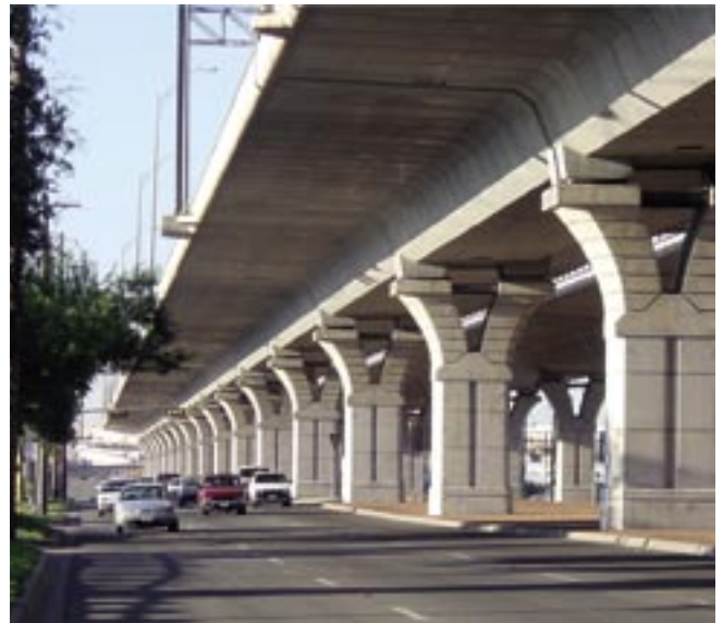
Fig. 14. U.S. 183 elevated viaduct.
