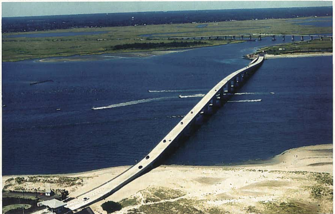
Fig. 19. Aerial photo of completed precast bridge with vehicular traffic viewed from the south Ocean City shore. Photo courtesy: Gregg Kohl, AC photo.
