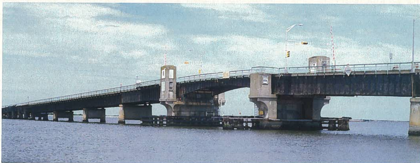
Fig. 2. The 75-year-old low-level steel bascule bridge was in imminent need of replacement.
