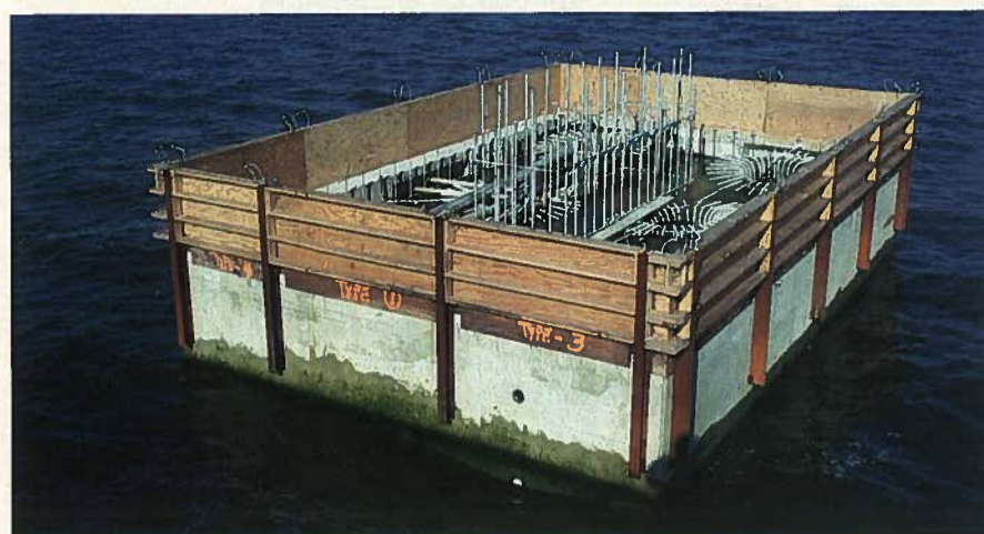
Fig. 7. Precast concrete cofferdam during construction of footing.
