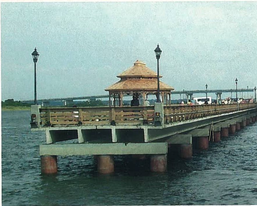
Fig. 3. A close-up of the historical restoration of a section of the old bridge as a fishing pier for local residents and tourists reveals an elegant precast concrete design. Photo courtesy: Gregg Kohl, AC Photo.
