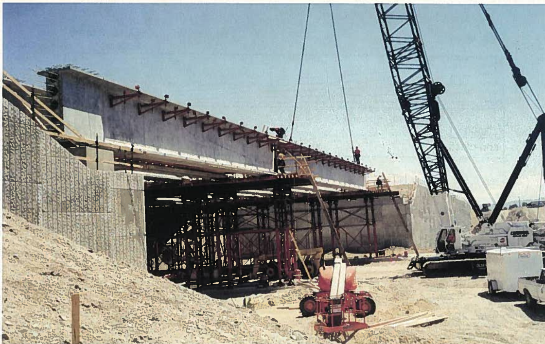
Fig. 1. Bridge over single-point urban interchange (I-15, Salt Lake City, Utah).
