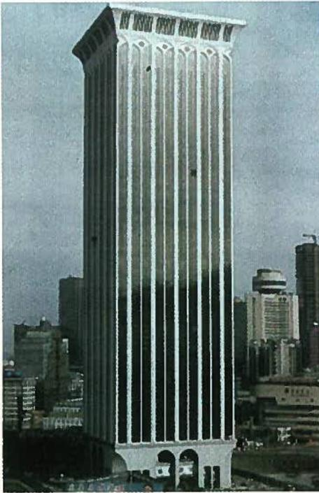
Fig. 6. Dalian Xiwang Building, Dalian City, China. The table below shows substantial savings in concrete and steel quantities by using precast/prestressed concrete technology. This building is located in a high seismic zone and, therefore, savings in materials will result in lower building dead weight and subsequently lower shear forces due to seismic loads.
