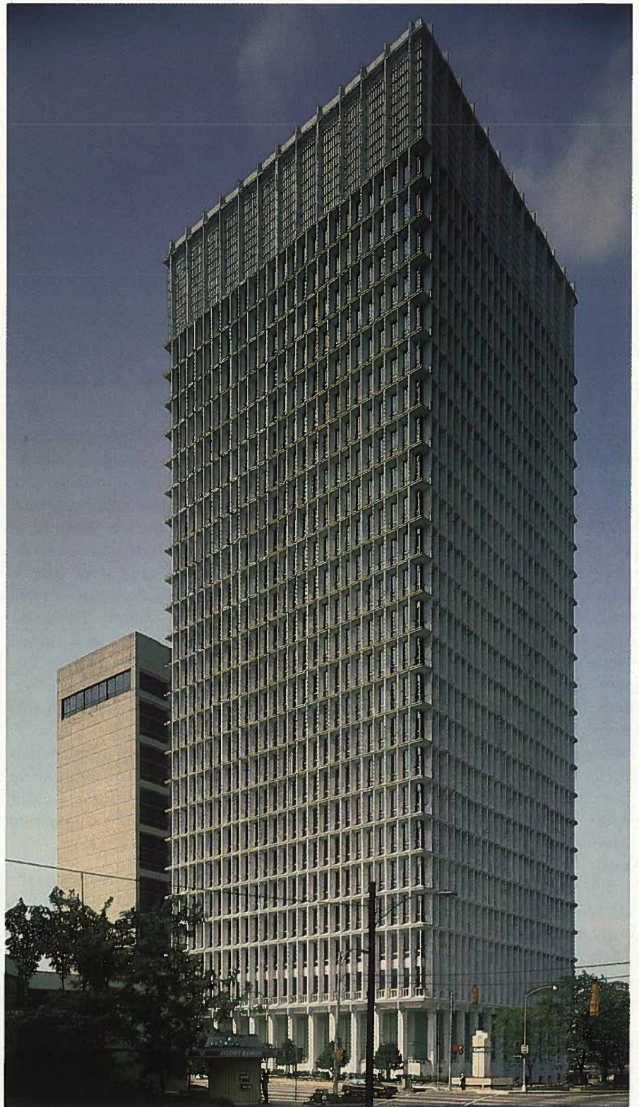
Fig. 1. The Georgia Center, Atlanta, Georgia, a 29-story building, was completed in 1964 and has 27 in. (690 mm) deep single window box units, each with 16 pieces of 1 in. (25 mm) marble veneer. Architects: Bodin and Lamberson; and Eggers and Higgins.
