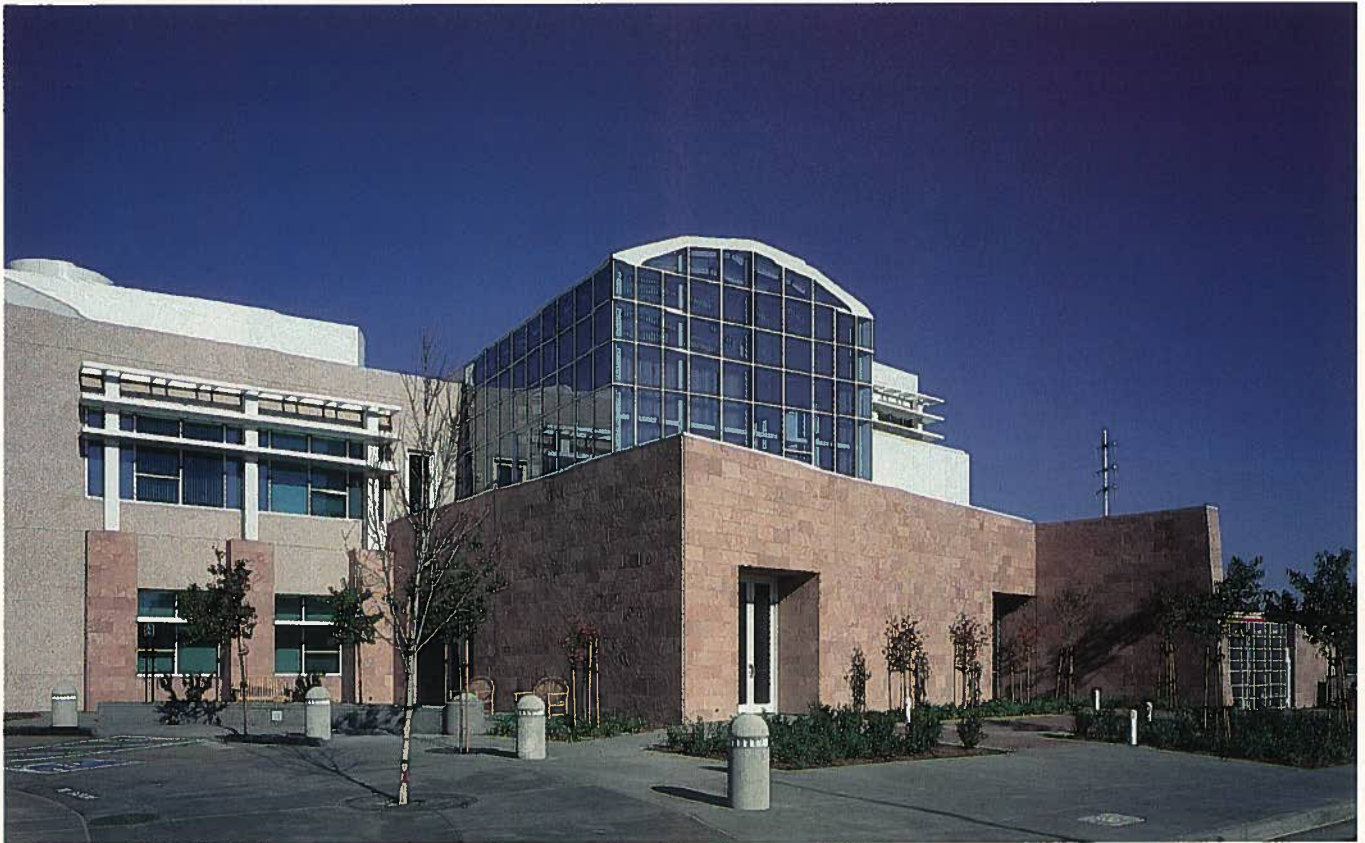
Fig. 24. Sacramento Municipal Utility District Customer Service Center, Sacramento, California. Architect: Williams + Paddon Architects & Planners/Inc., Roseville, California.
