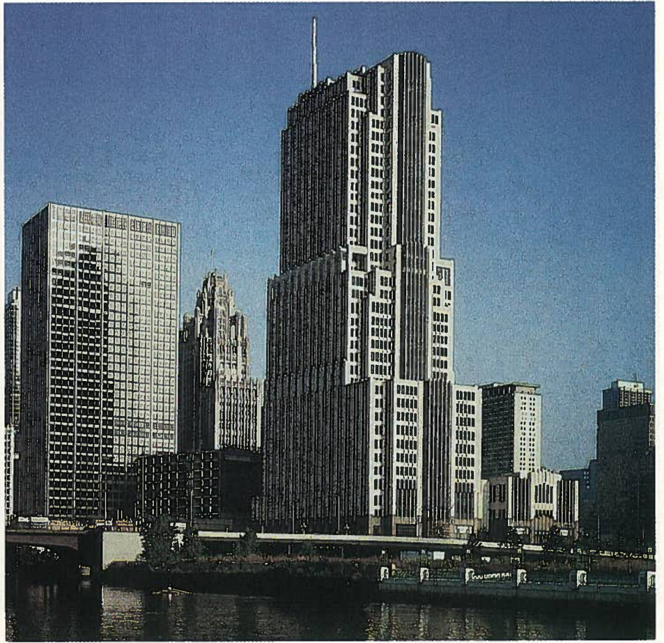
Fig. 29. NBC Tower at Cityfront Center, Chicago, Illinois. Architect: Skidmore, Owings, & Merrill, Chicago, Illinois.
