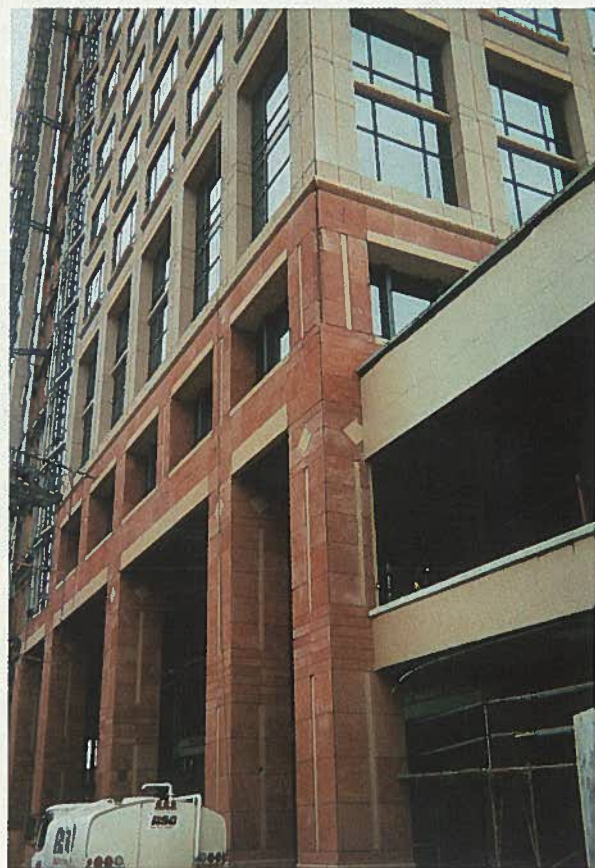
Fig. 23(b). Closeup of completed lower story panels.
