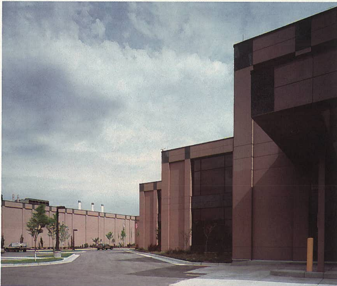
Fig. 32. Mountain Fuel North Service Center, Salt Lake City, Utah. Architect: Richardson Companies, Salt Lake City, Utah.
