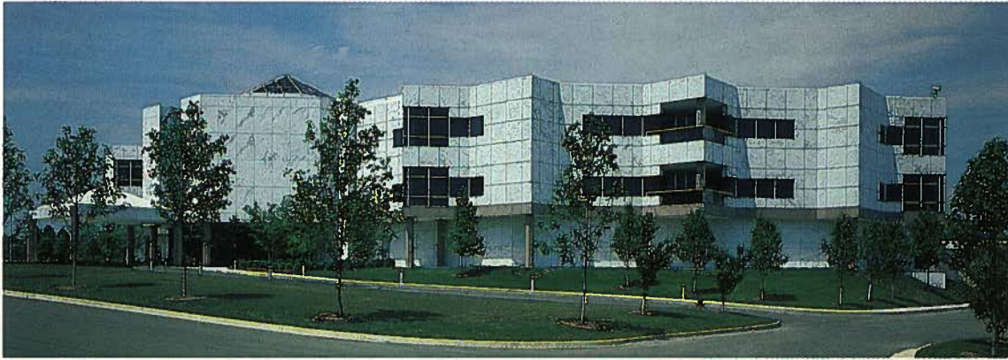
Fig. 18. Hospital Corporation of America Data Center, Nashville, Tennessee. Architect: Gresham, Smith and Partners, Nashville, Tennessee.
