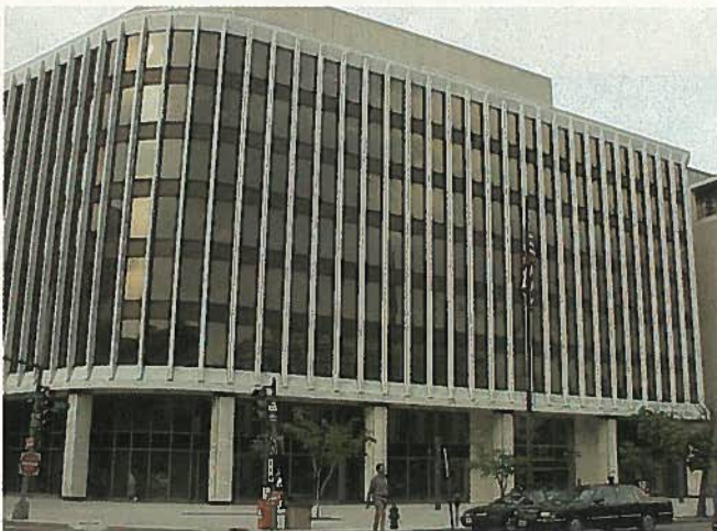
Fig. 21(a). Airline Pilots Association Headquarters, Washington, D.C. Architect: Vlastimil Koubek, Washington, D.C.
