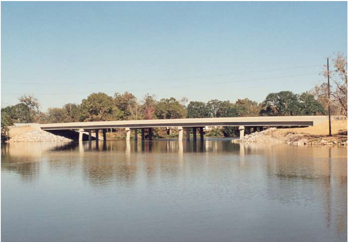
Fig. 6. The use of HPC allowed the bridge engineers to eliminate one girder line thus saving on the cost of the superstructure.
