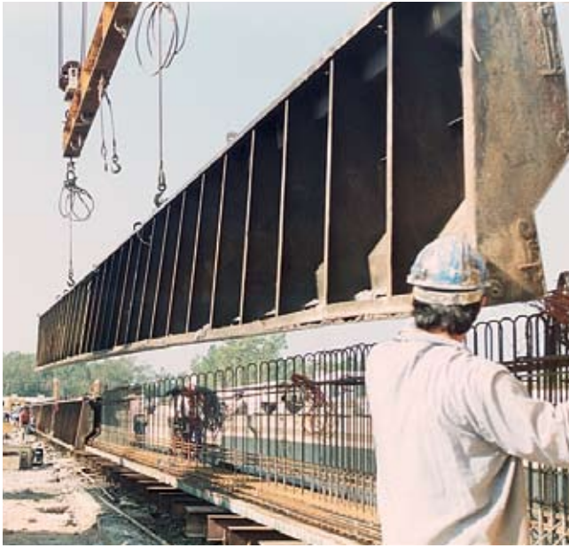
Fig. 10. Readyng forms for casting girder.
