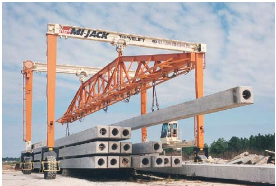
Fig. 5. Newly cast piles being stacked at precaster's yard.
