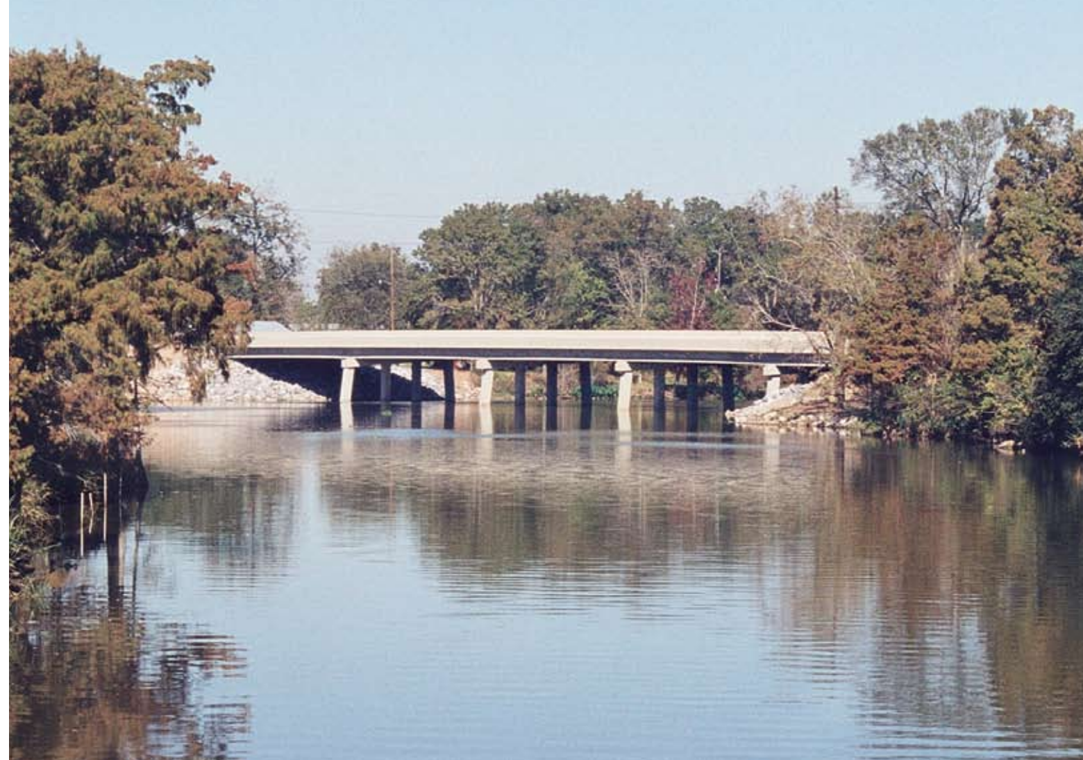
Fig. 1. The Charenton Canal Bridge, Charenton, Louisiana. The 365 ft (111 m), five-span precast, prestressed concrete structure demonstrates the effectiveness of using HPC.
