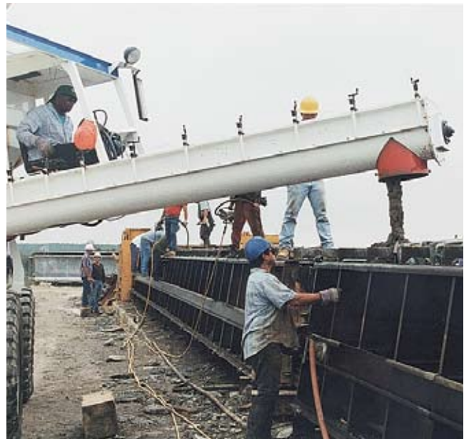
Fig. 11. Concreting operation for casting girder.
