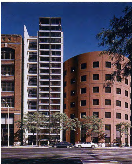
Fig. 46a. Jefferson Avenue Parking Structure, Detroit, Michigan.
