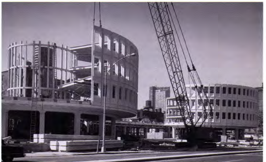
Fig. 6. Three-story panels supporting double tees.
