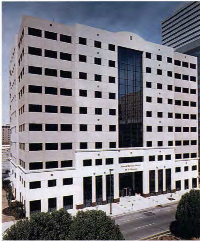
Fig. 41. Internal Revenue Service office building, Oklahoma City, Oklahoma.
