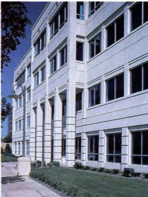
Fig. 42a. The Crescent Town Center Campus in Denver Technological Center, Denver, Colorado, features a series of buildings designed around an open, park-like crescent.
