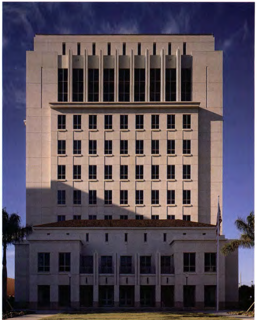
Fig. 11. Shear wall at the corners of the Sarasota County Judicial Center, Sarasota, Florida.
