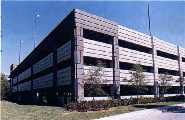
Fig. 38. Barnett Bank parking facility, Jacksonville, Florida.
