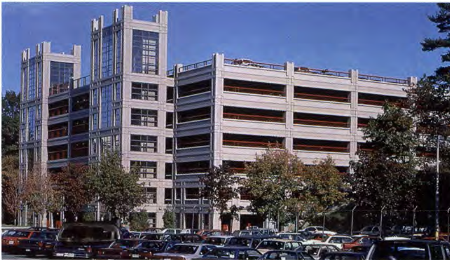
Fig. 37a. The Boston College parking structure in Chestnut Hill, Massachusetts.
