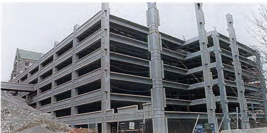
Fig. 37b. Early construction shot of the Boston College parking structure.
