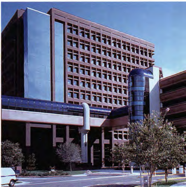
Fig. 44. Loadbearing window boxes on Orange County Regional Service Center, Orlando, Florida.
