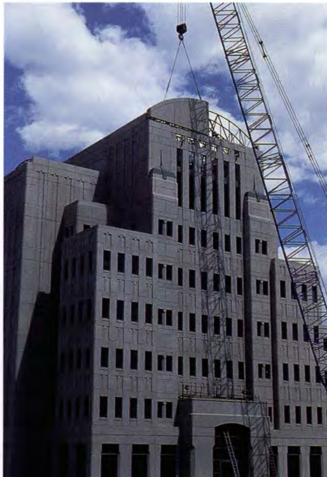
Fig. 47c. Final erection shot of Denver Wastewater Management Building, Denver, Colorado.
