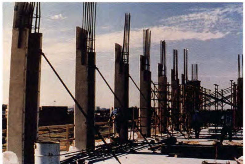
Fig. 21. Panels serve double duty as formwork for columns and perimeter beams.
