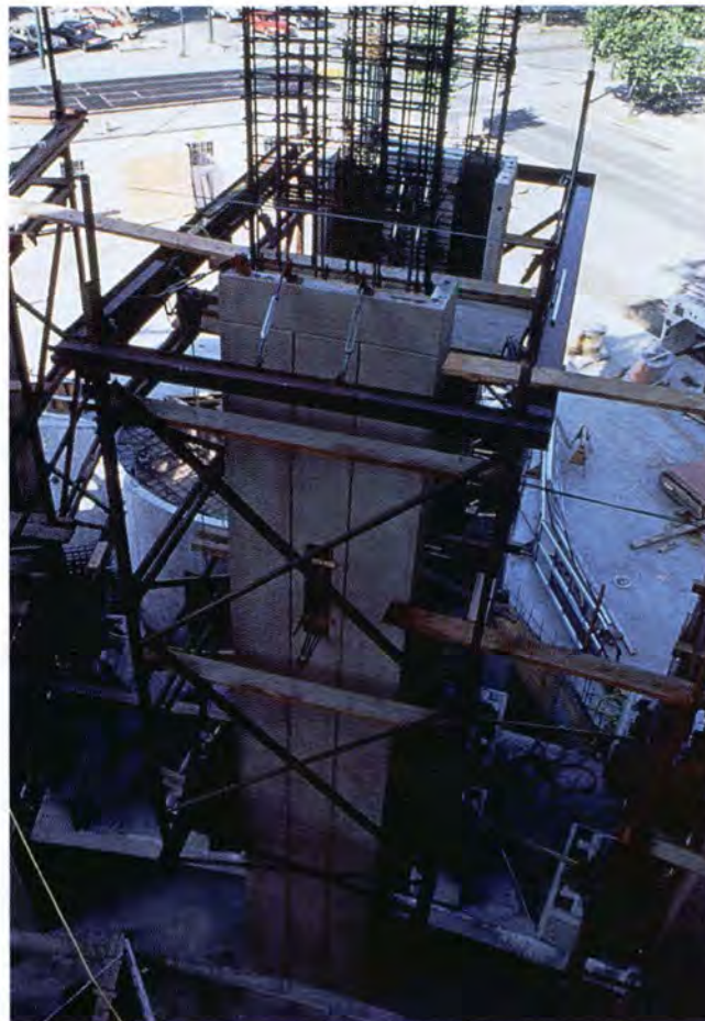
Fig. 17. Panels serve as forms for cast-in-place concrete.
