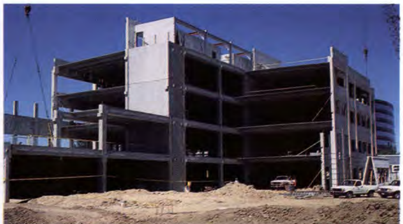
Fig. 42b. The use of integrated loadbearing/architectural spandrel panels erected in 8 weeks facilitated a tight construction schedule (The Crescent Town Center Campus, Denver, Colorado).
