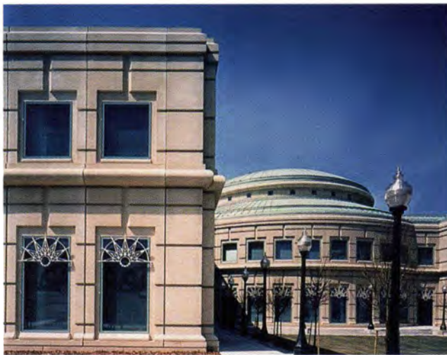
Fig. 45b. Details on loadbearing panels for Aurora Municipal Justice Center, Aurora, Colorado.
