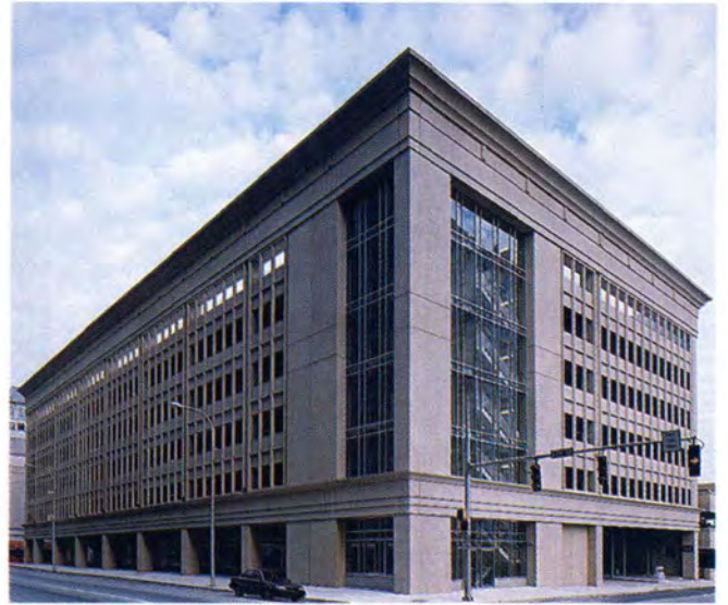
Fig. 39. Community Service Building Garage, Wilmington, Delaware.
