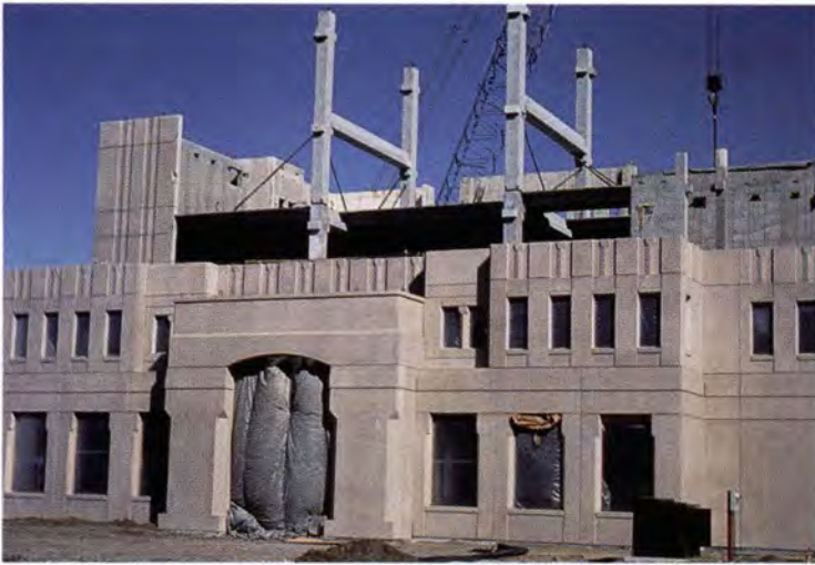
Fig. 47a. Construction of total precast Denver Wastewater Management Building, Denver, Colorado.
