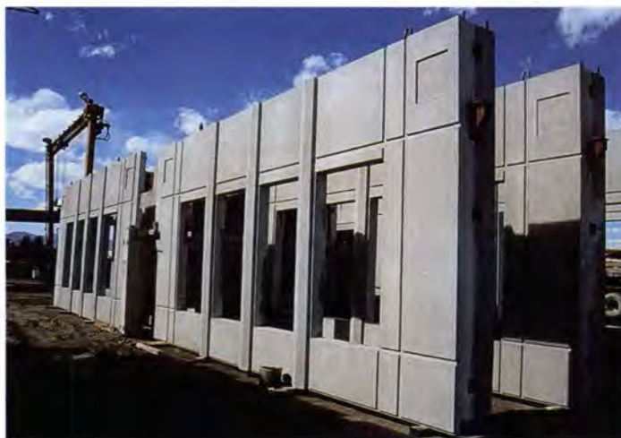
Fig. 3. Single-story wall panels.
