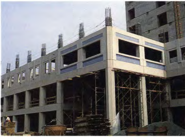
Fig. 18. Construction of Marathon Plaza, San Francisco, California.
