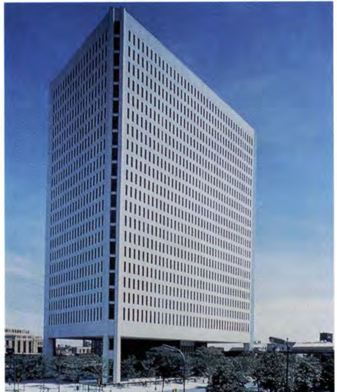
Fig. 35. Window wall panels serve as elements of Vierendeel truss on One Hundred Washington Square office building, Minneapolis, Minnesota.
