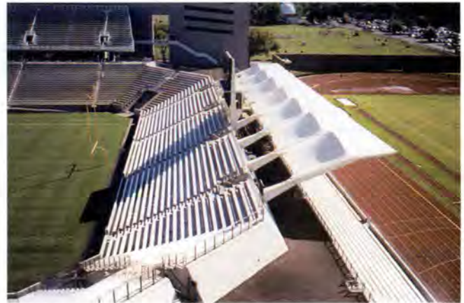
Fig. 18. The adjoining track stadium features precast concrete seating covered with a fabric canopy held in place by cantilevered steel posts.
