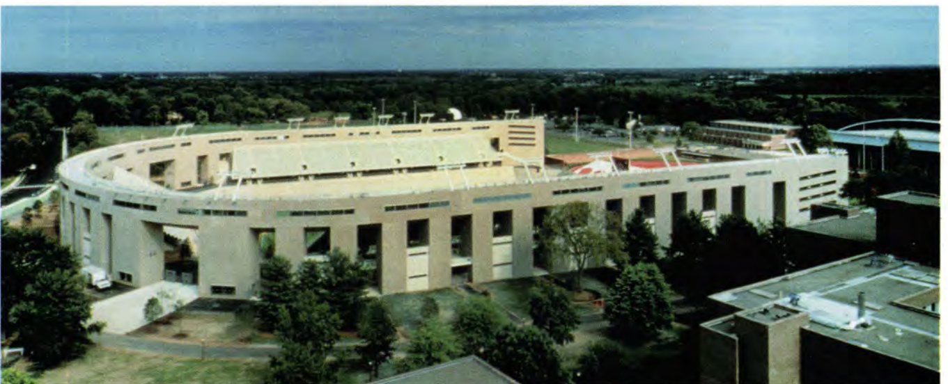
Fig. 2. Overview shows how the horseshoe-shaped stadium connects visually to the track stadium at its open end and further along to the 1960s gymnasium at the far right.
