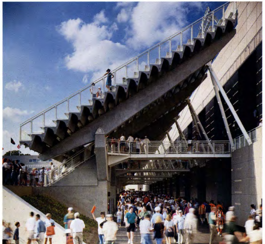
Fig. 11. Overview of grandstand with concourse below. The risers were designed to "float" above the bowl level and allow daylight to enter the concourse.
