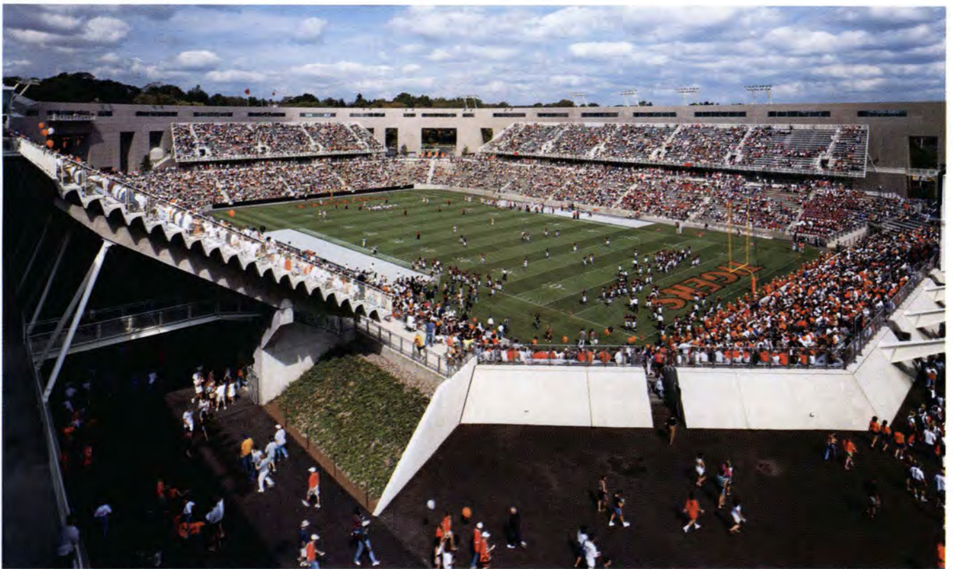
Fig. 1. Princeton University Stadium features several unique aspects including trapezoidal upper seating on three sides made of precast concrete triple risers and a perimeter building housing all services that remains open year-round, as does the colonnade behind the seating sections.
