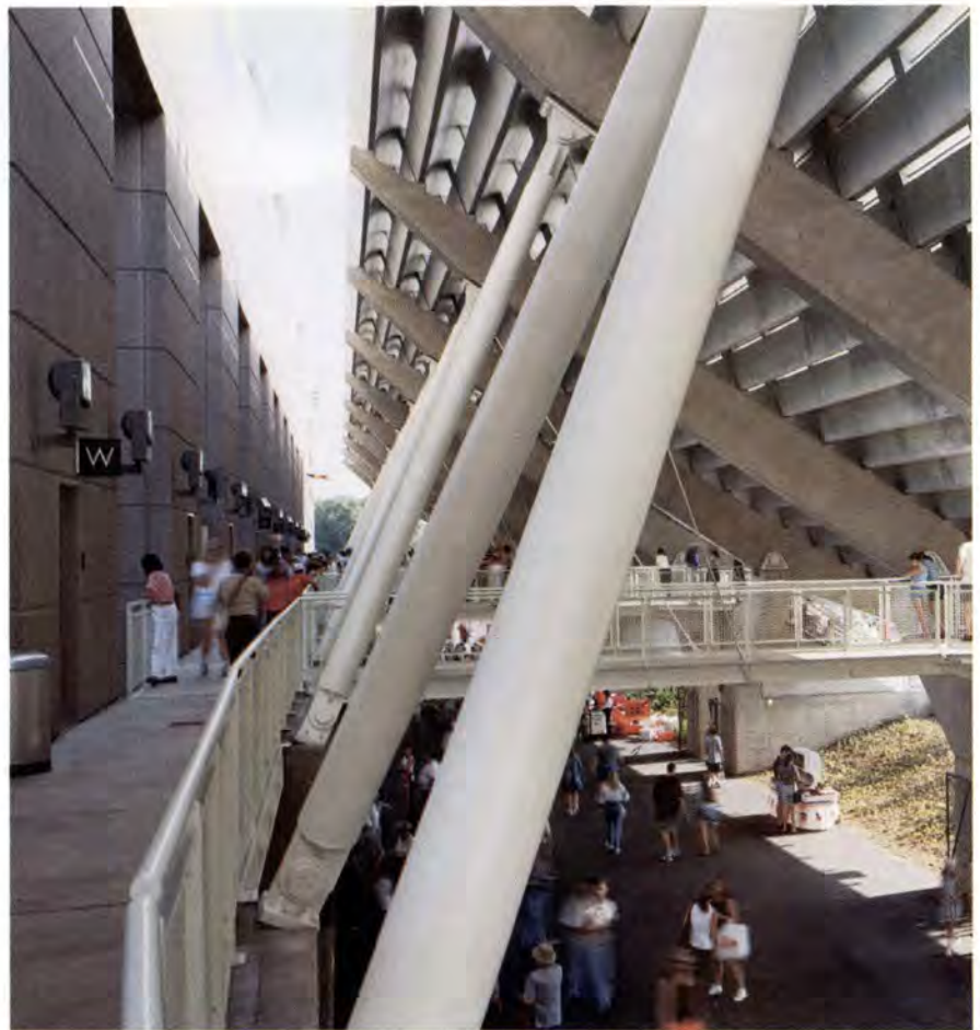
Fig. 14. Looking down into concourse. In background, risers and raker beams are visible. In foreground, base connections of steel posts to walls can be seen.
