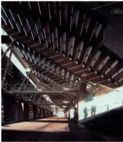
Fig. 13. Overview of concourse showing underside of risers allowing light to penetrate.
