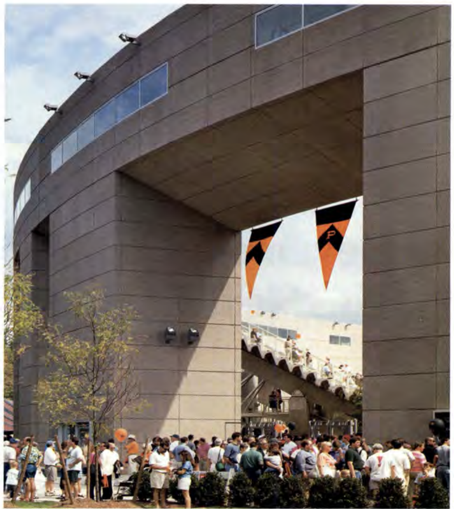
Fig. 20. Main entrance of stadium. A heavy sandblasted finish was applied to the building's panels to help tie its look to the site's original concrete stadium.
