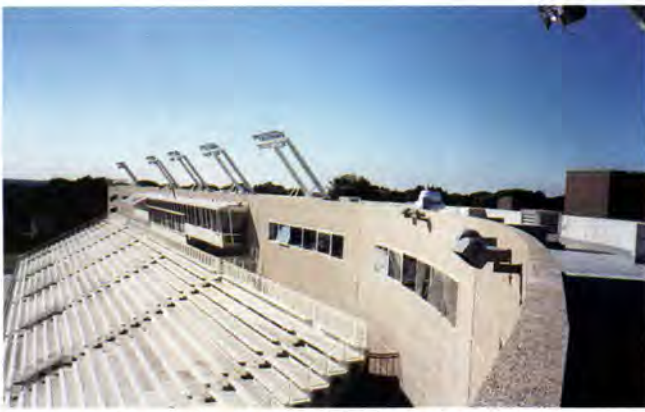
Fig. 17. Although the corners of the horseshoe-shaped building appear to curve, the panels were in fact faceted on their face to allow them to remain flat while making the two required curves.
