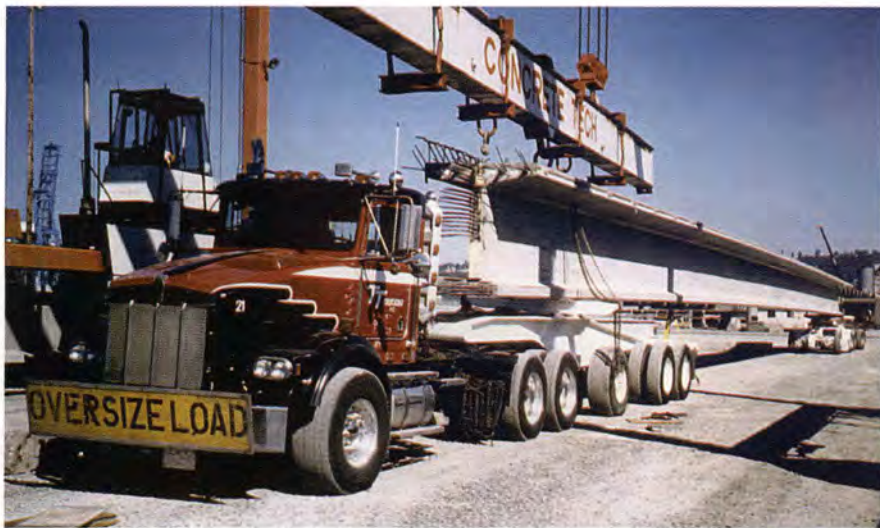
Fig. 26. 168 ft (51.2 m) long, 180,000 lb (81648 kg) decked bulb-tee girder.
