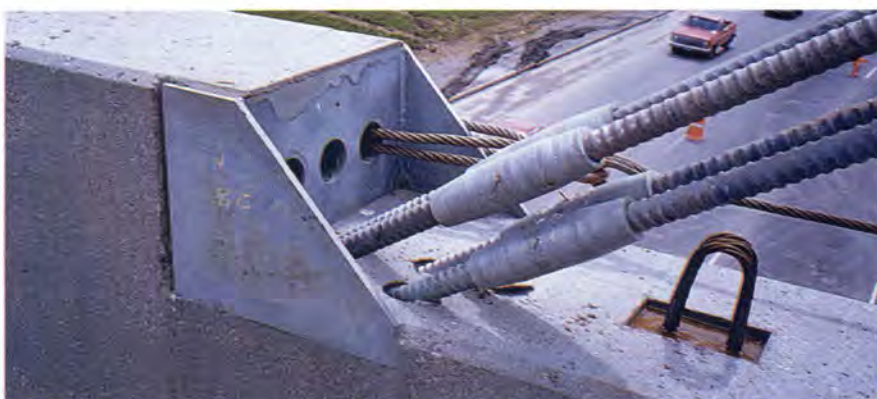
Fig. 8. Bridge deck stay connection.
