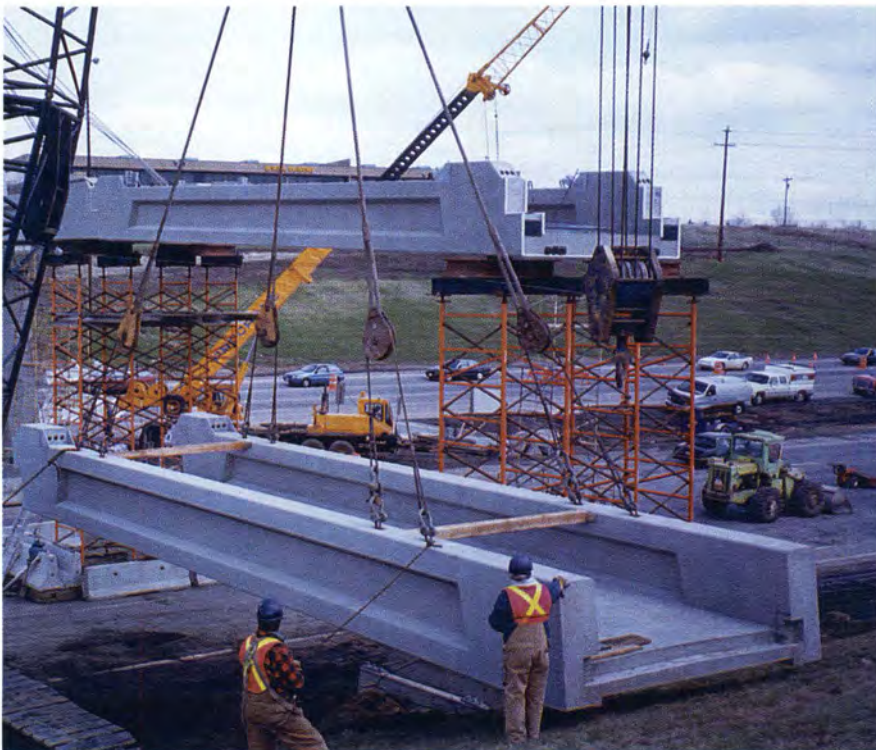
Fig. 6. Erection of last bridge deck component on west span.
