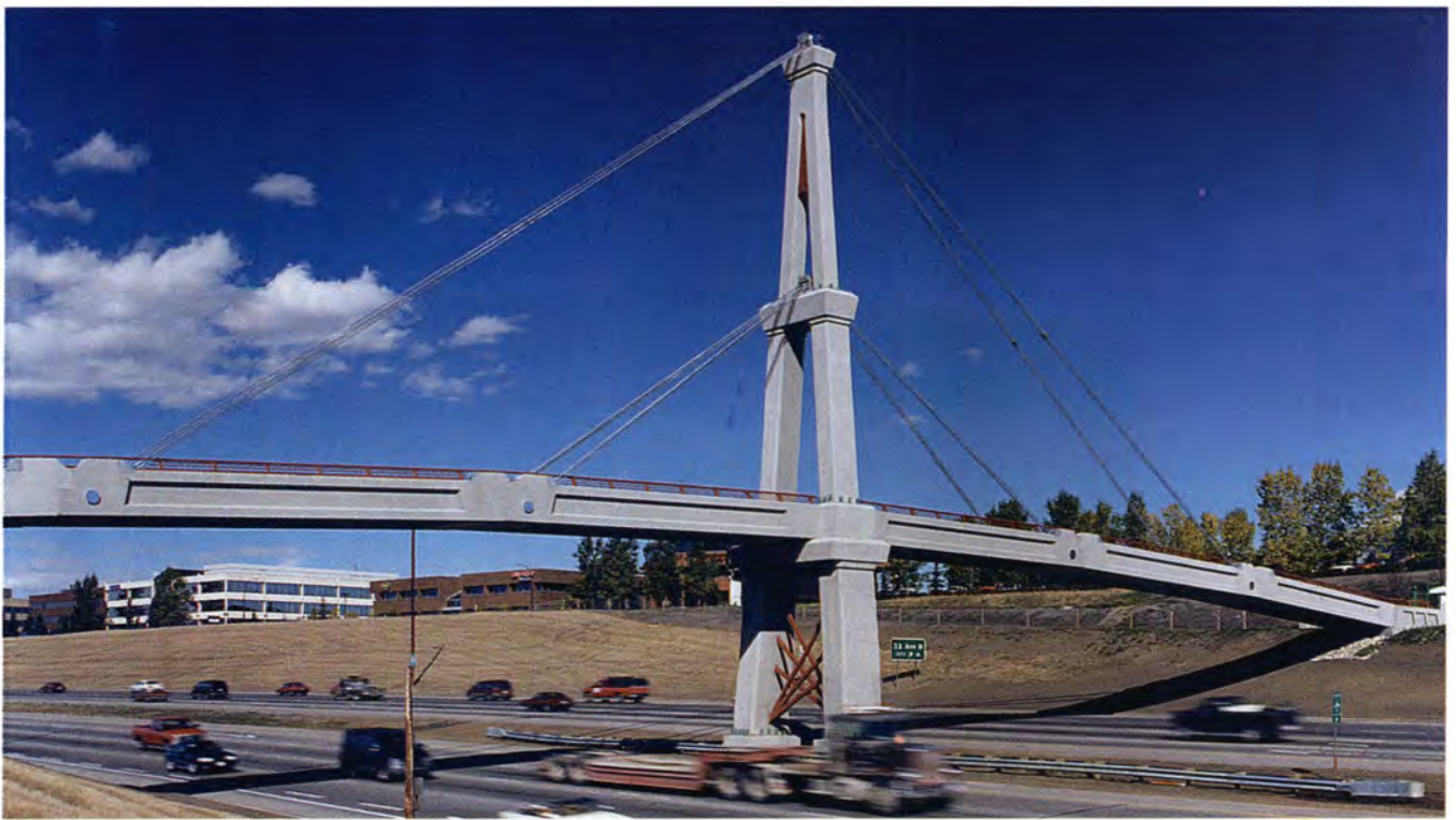
Fig. 9. Completed bridge looking toward the northeast.
