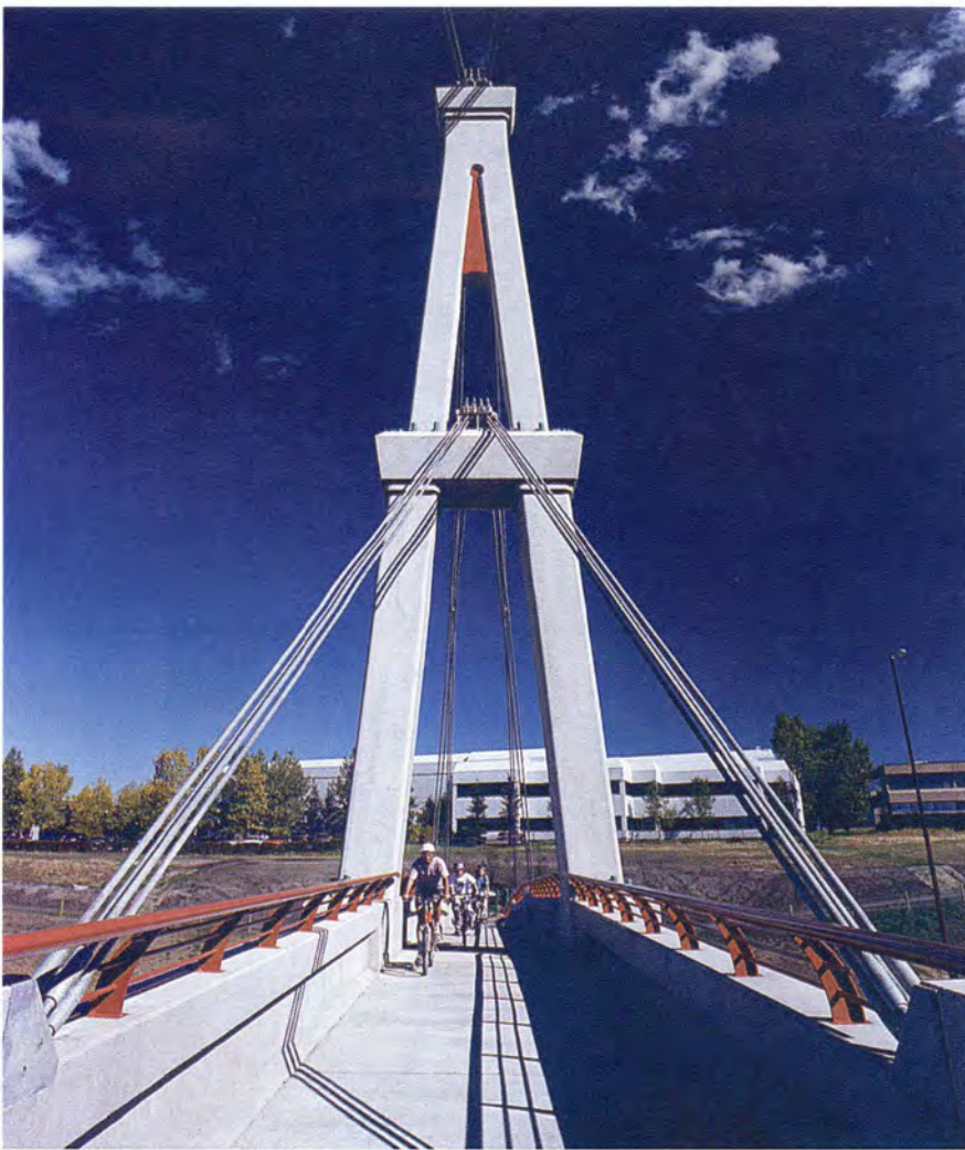
Fig. 11. Completed bridge looking toward the east along the length of the bridge.
