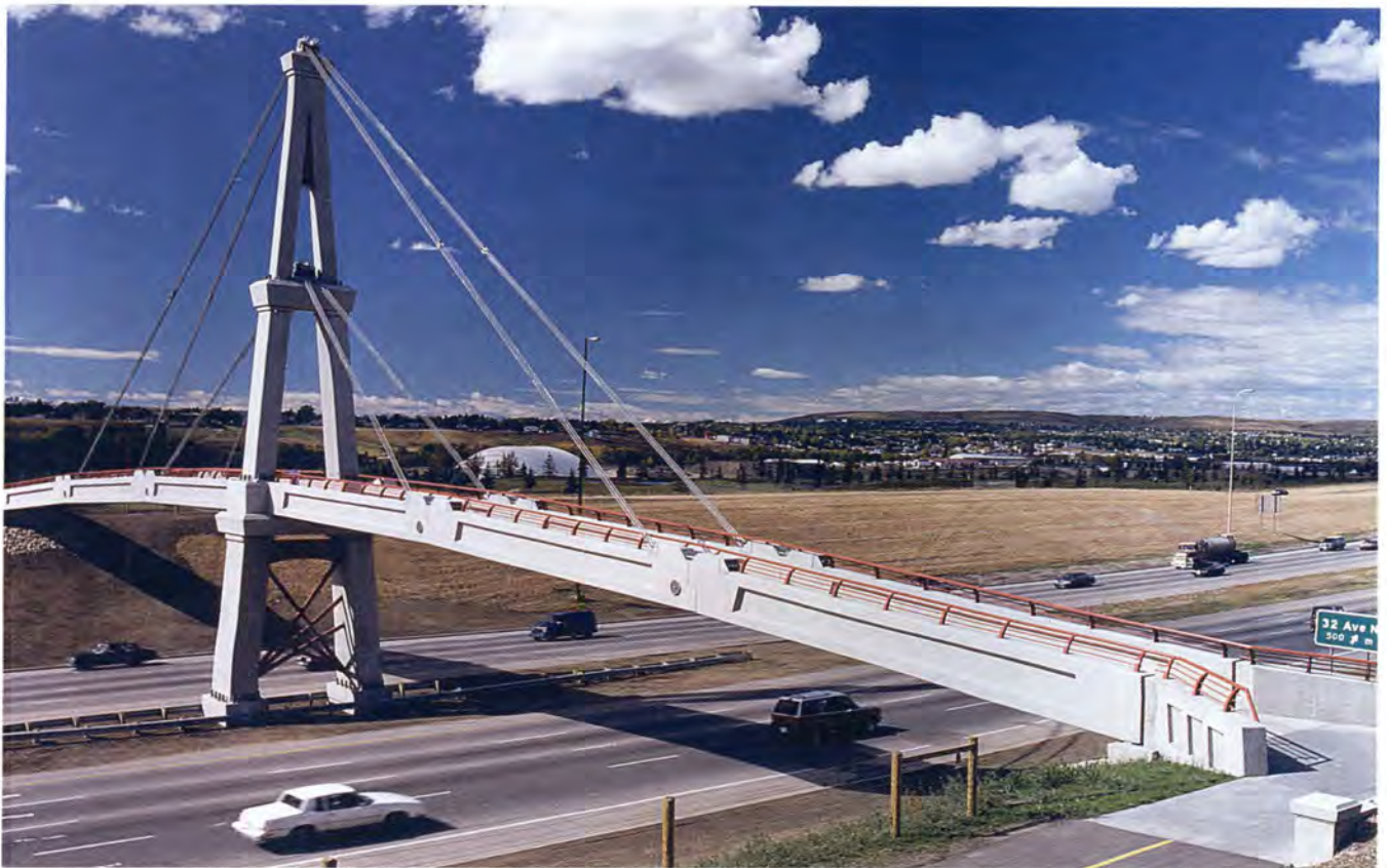
Fig. 1. Fox Hollow Pedestrian Bridge, Calgary, Alberta, Canada (looking toward northeast).
