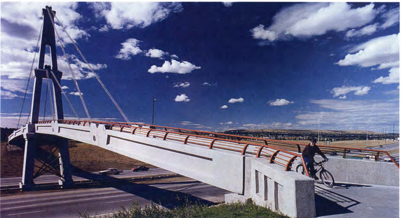
Fig. 12. Completed structure looking at the east abutment.
