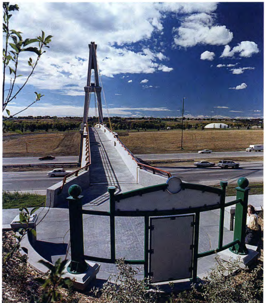
Fig. 10. Completed structure looking toward the west from the east abutment.
