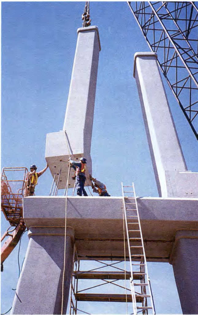
Fig. 4. Erection of upper tower column.
