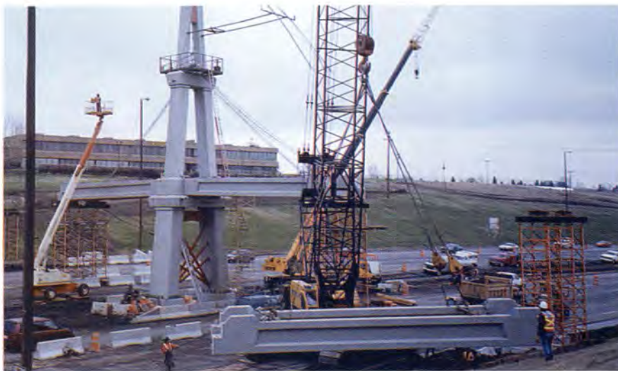
Fig. 7. Erection of bridge deck components.
