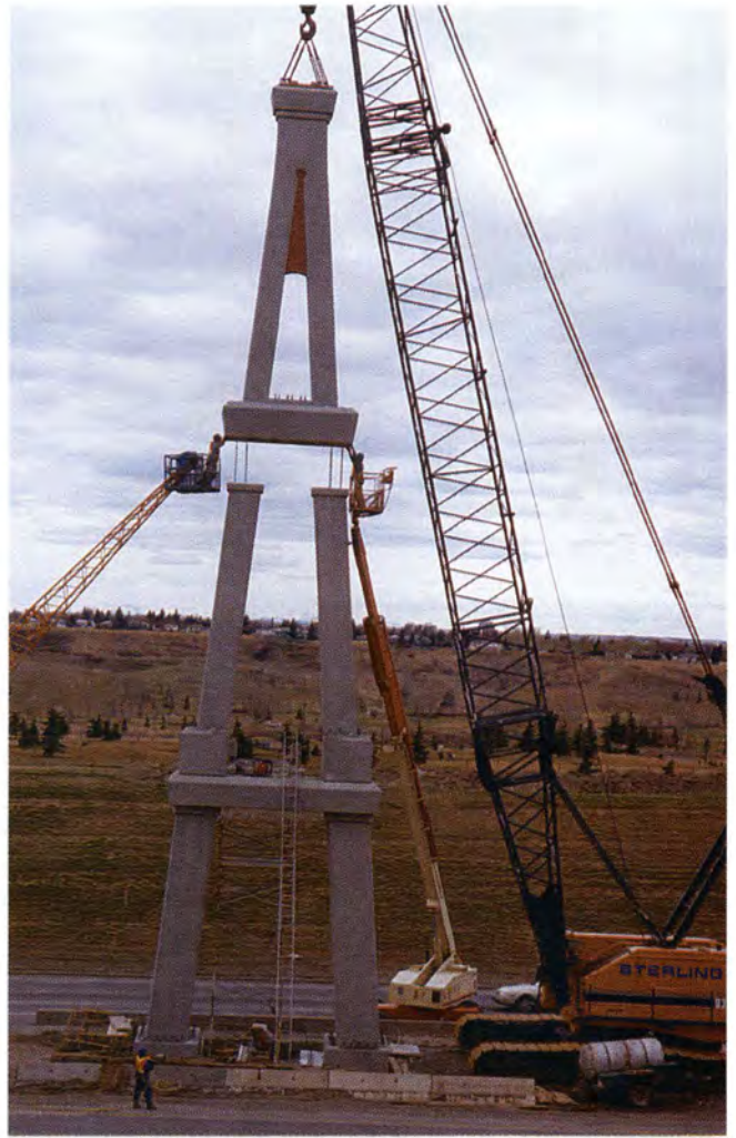
Fig. 5. Erection of tower A-frame.
