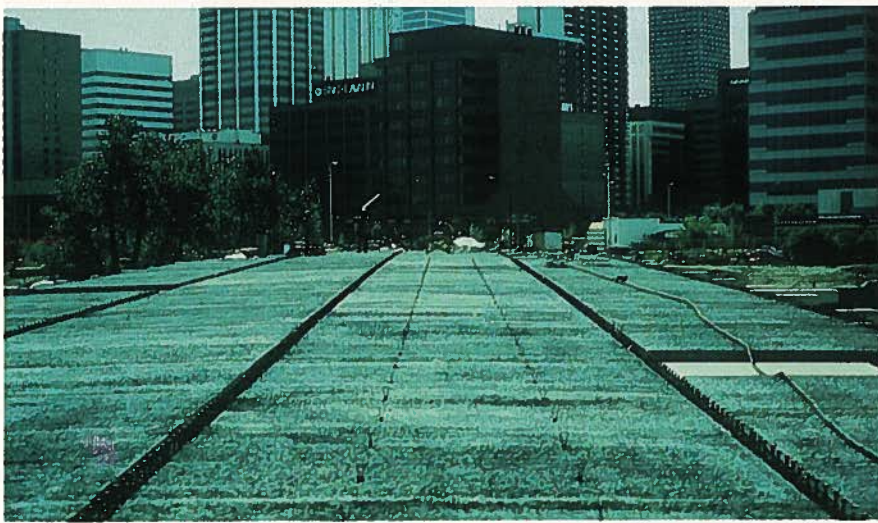
Fig. 11. Precast deck panels in place.
