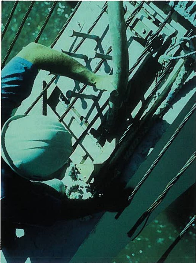
Fig. 9. Installing bearings at precast bracket locations.
