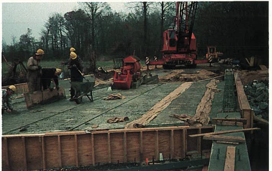
Fig. 5. Grouting of slab joints prior to overlay placement.
