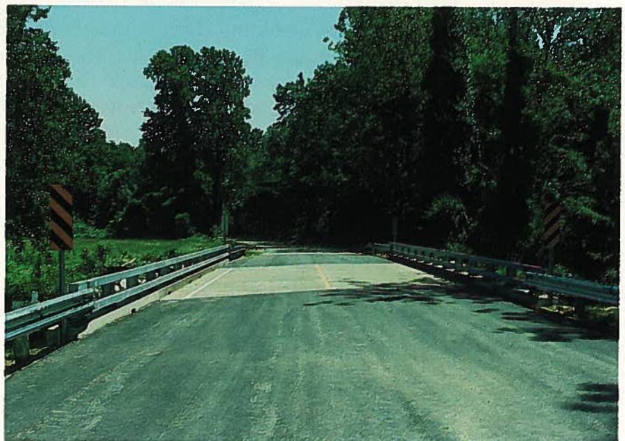
Fig. 7. Completed structure on Maryland Route 404 over Norwich Creek.
