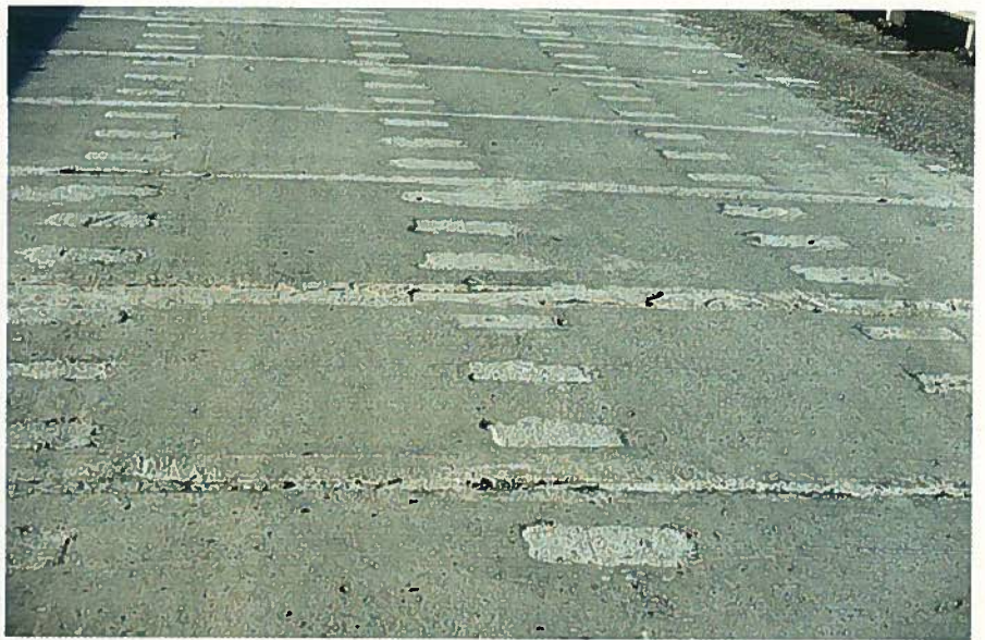
Fig. 34. Typical overview of deck panels, Dalton Highway Bridges, Alaska.
