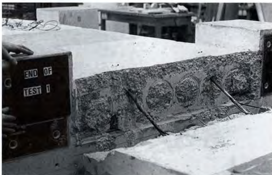
Fig. 14a. The end of Test B on connection Type 1; failure region.
