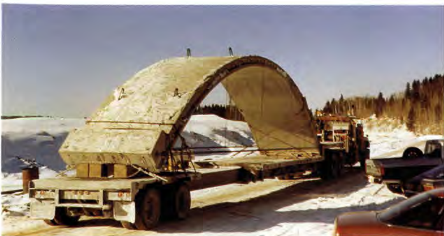
Fig. 12. Trucking of arch segment.
