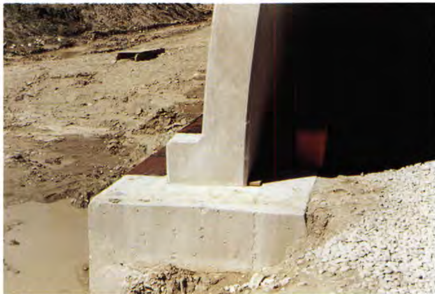
Fig. 14. Arch segment grouted into footing pedestal.
