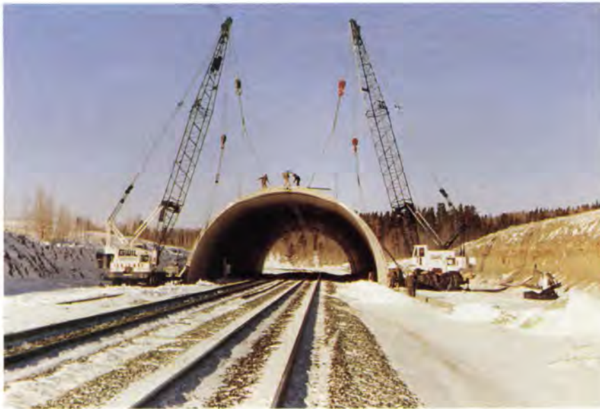
Fig. 13. Erection of arch segments.
