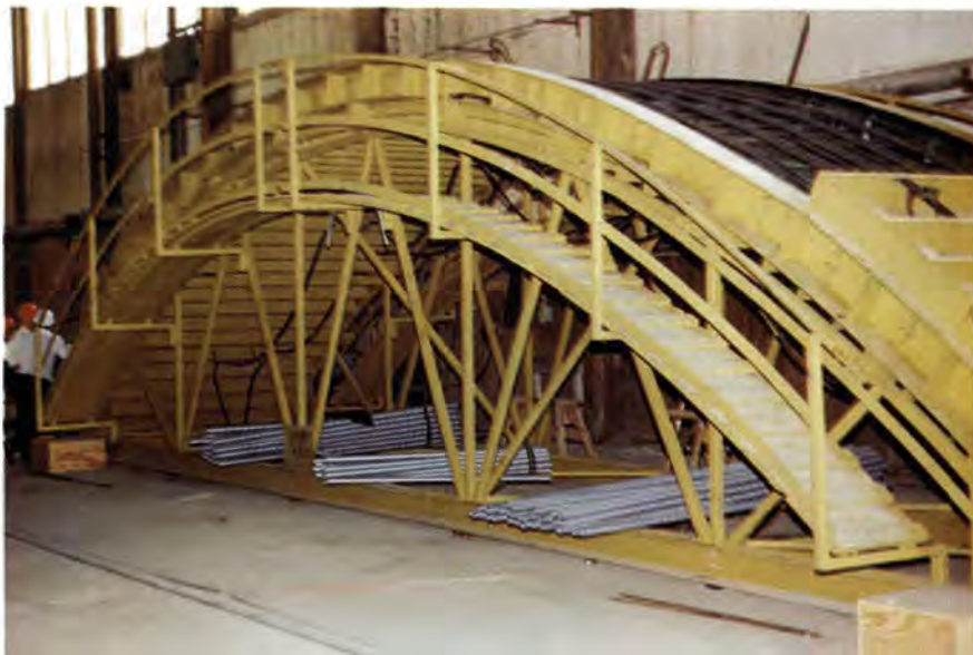
Fig. 11. Form for arch segments.
