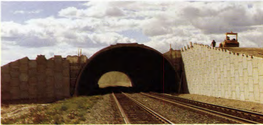
Fig. 16. Backfilling of arch.
