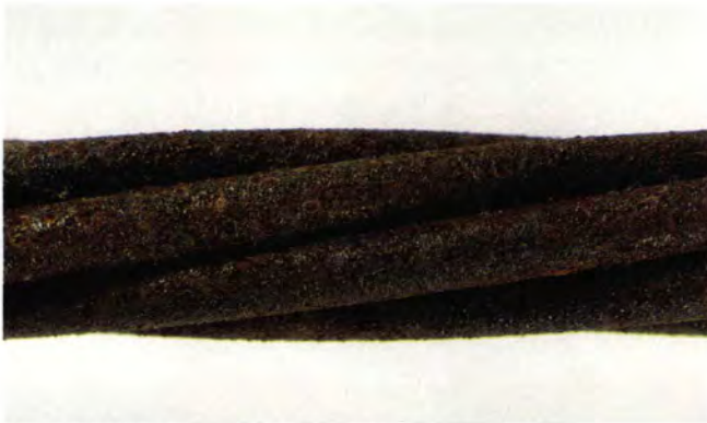
Photo 7. Strand surface before cleaning.
