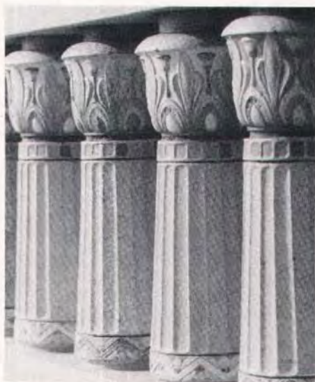
Close-up view of terra cotta balusters.
