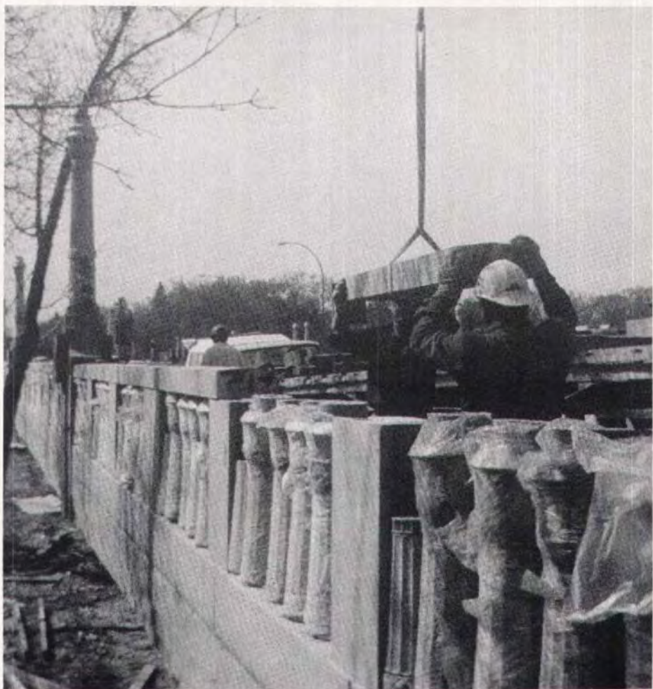
Installation of precast top rail unit.
