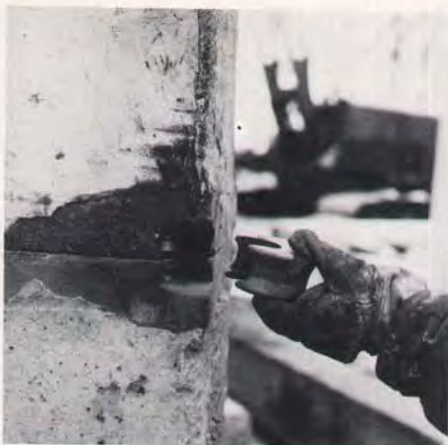
Inserting wedges to connect the piles.
