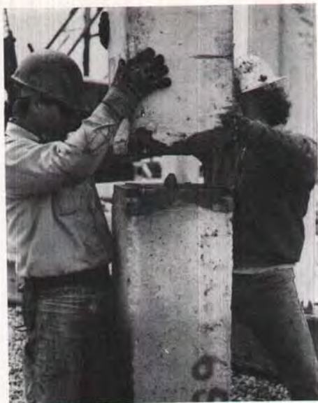
Aligning two piles prior to splicing.
