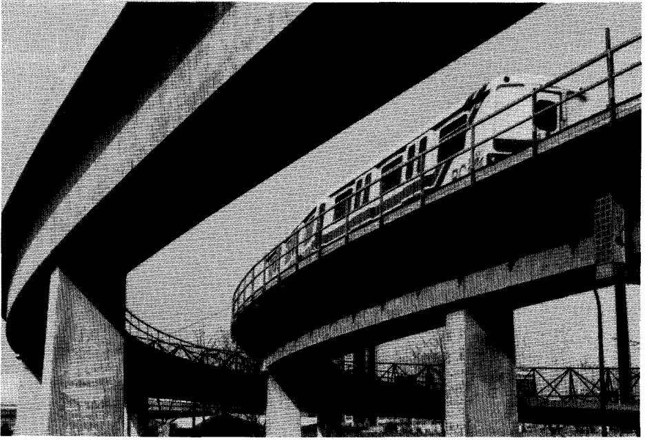
Fig. 31. Finished portion of the aerial guideway for Vancouver ALRT project.
