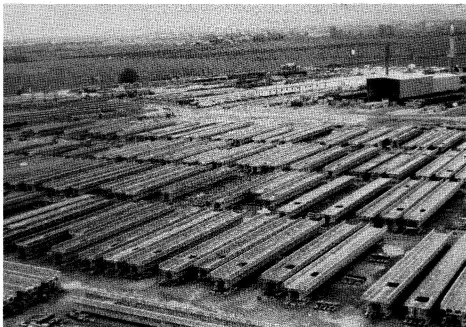
Fig. 18. Portion of beam storage yard.
