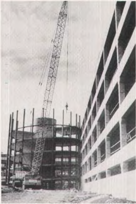
Fig. 17. Erection of spiral ramp.
