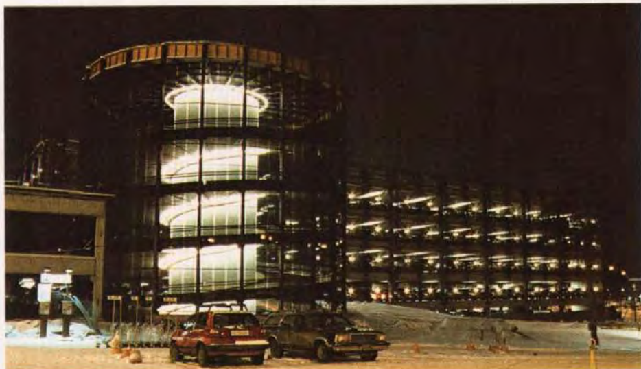
Fig. 1a. Spiral ramp at night with main parking structure in background.
