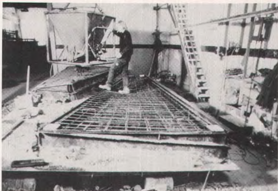
Fig. 12. Casting of prefabricated panels.
