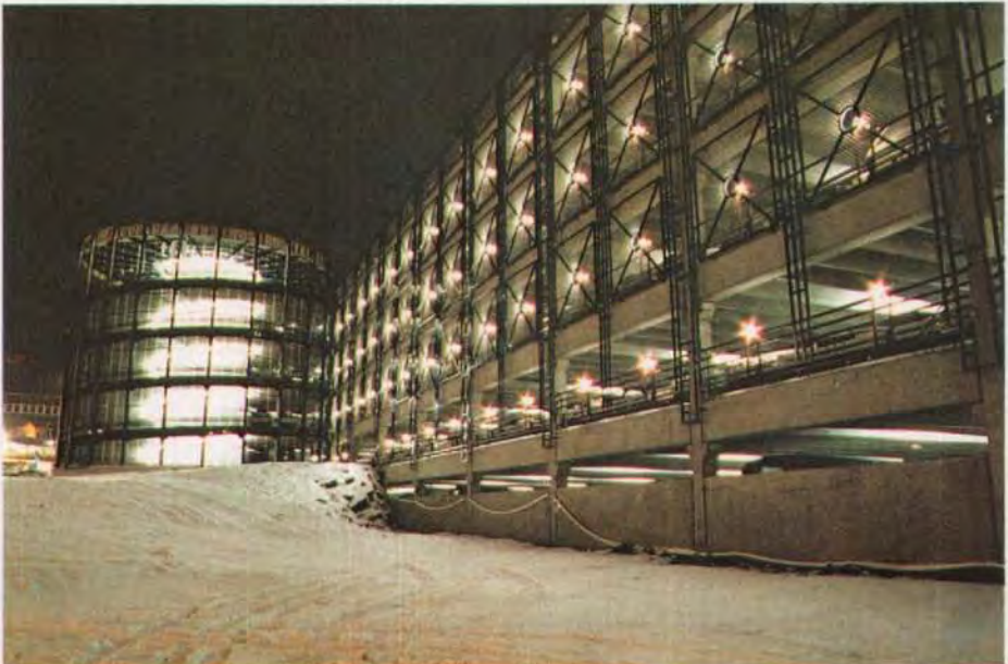
Fig. 19. Shot of spiral ramp and main parking structure on a winter night.
