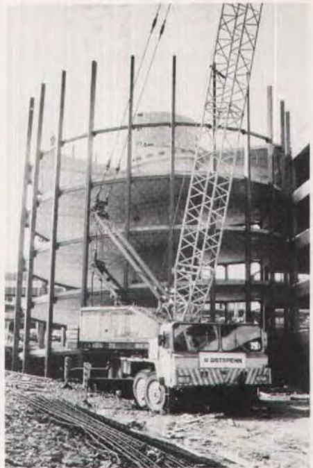
Fig. 18. Closeup of spiral ramp.
