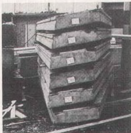
Fig. 9. Stack of panels.
