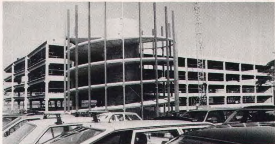
Fig. 20. Overall view of spiral ramp and main parking structure nearing completion.
