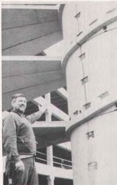
Fig. 14. Proud foreman showing perfect fit of components of spiral ramp.
