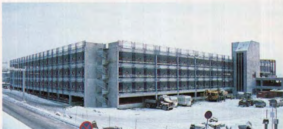
Fig. 1b. Overall view of parking structure on a winter day.
