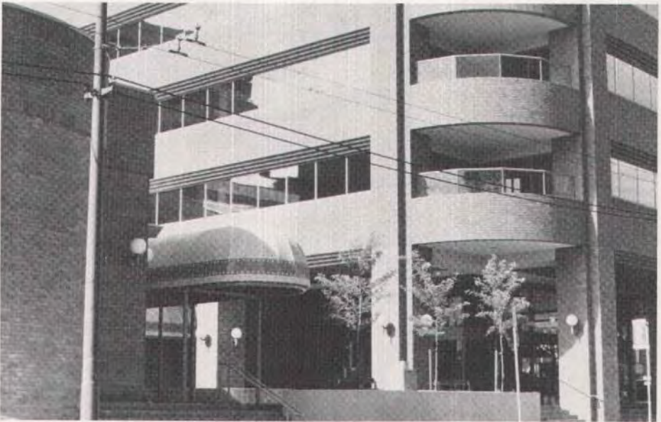
Fig. 5. Office building, 1125 Howe St., Vancouver, British Columbia. Architect: Eng and Wright Partners, Vancouver.
