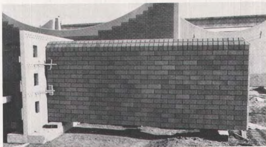
Fig. 15. Vertical easels can also be an effective restraint for stockpiling.
