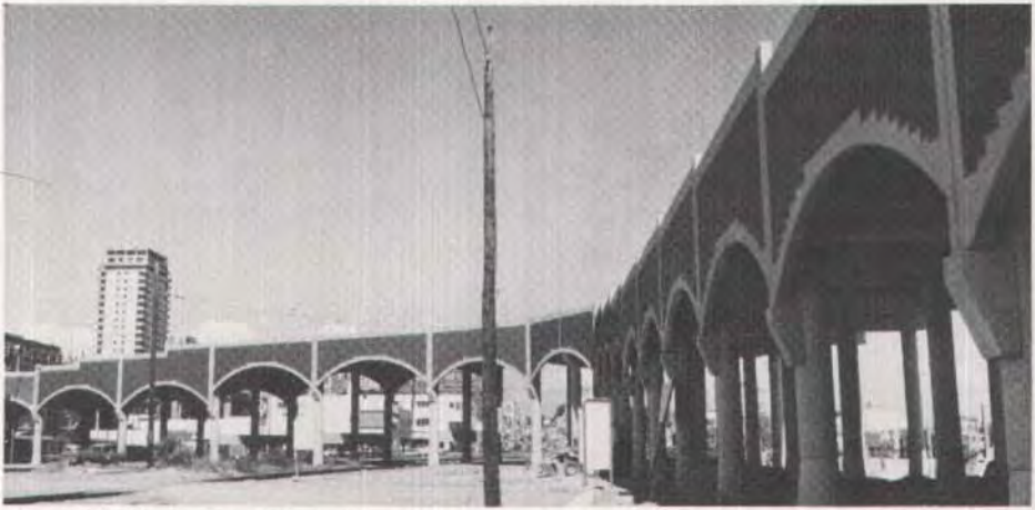
Fig. 4. McGinnis Road Overpass, New Westminster, British Columbia. Architect: John Moore, Vancouver.
