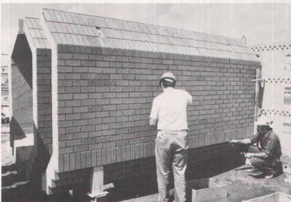
Fig. 17. Removal of rubber formers and cosmetic finishing is completed in the first 24 hours after stripping.
