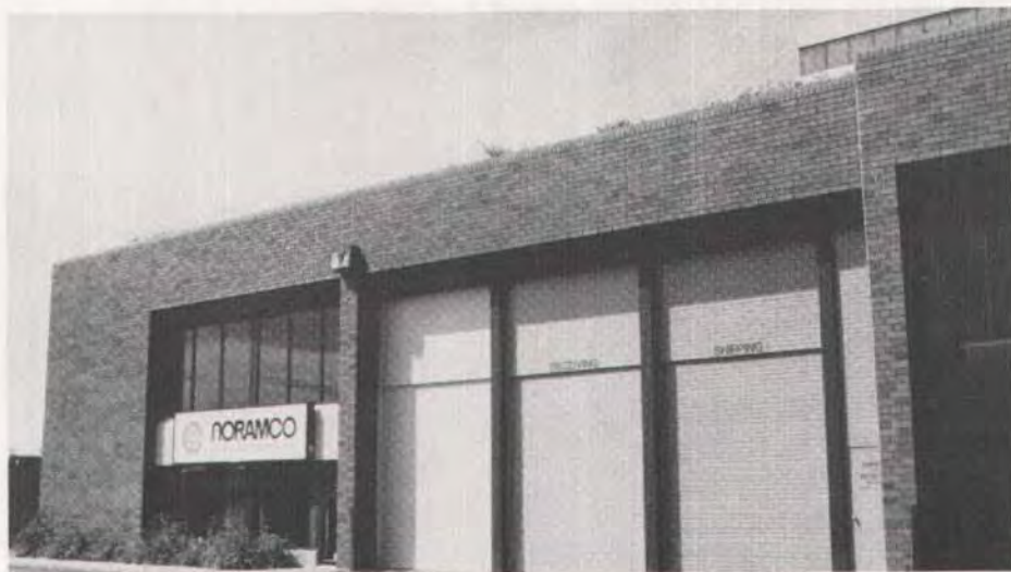
Fig. 3. Commerce Court, Lougheed Highway, Vancouver, British Columbia. Architect: Raymond Letkeman, Vancouver.
