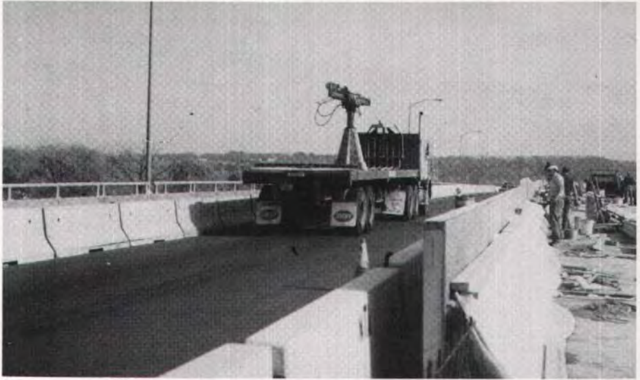
Fig. 29. Connecticut River Bridge, Massachusetts Turnpike Authority.
