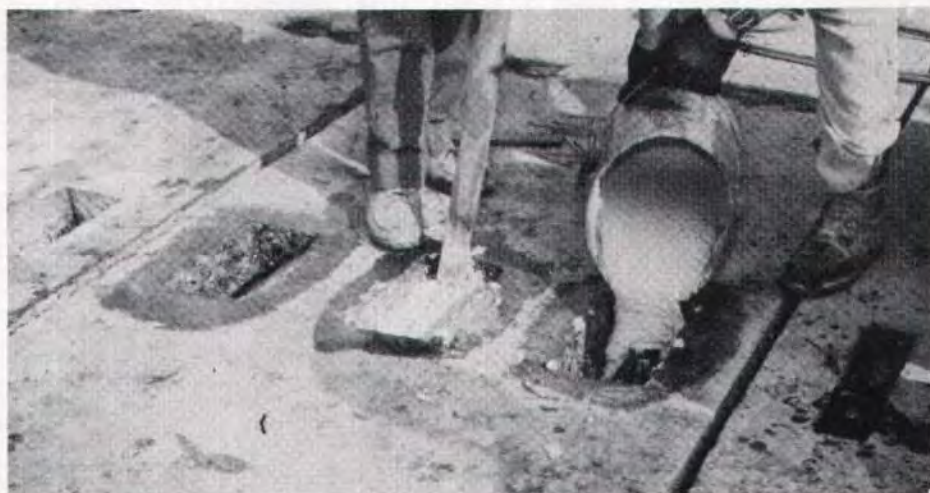
Fig. 15. Casting of epoxy mortar in shear pocket (NYSTA).
