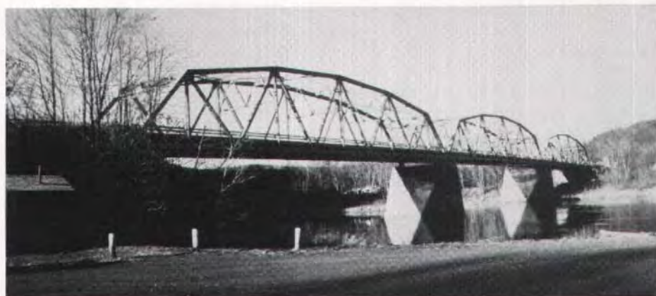
Fig. 35. Bridge No. 6 over Delaware River, NYSDOT.
