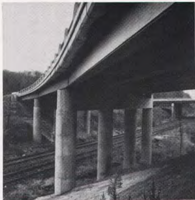
Fig. 22. Harriman Interchange Ramp Bridge, NYSTA.
