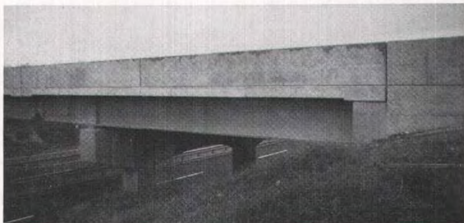
Fig. 26. Quakertown Interchange Bridge, Pennsylvania Turnpike Commission.
