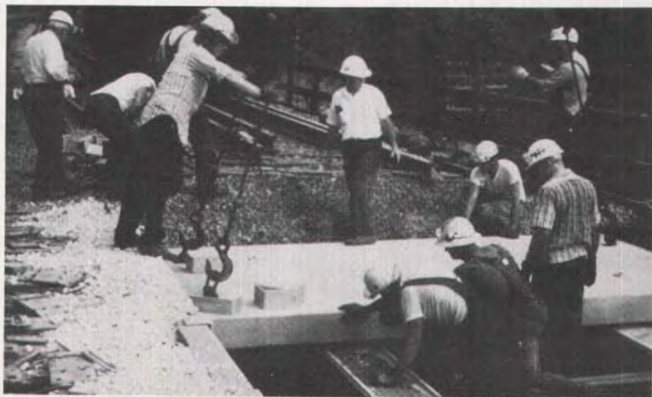
Fig. 59. Precast slab placement, Santa Fe Railway.
