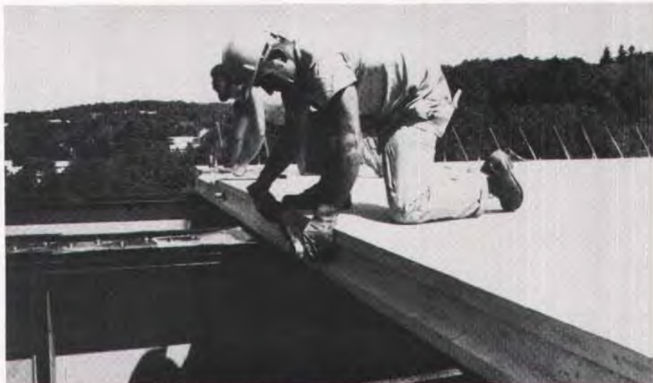
Fig. 25. Longitudinal post-tensioning (Clark Summit Bridge).
