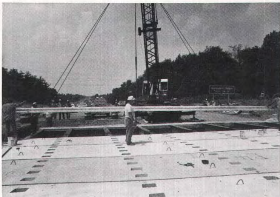
Fig. 20. Placement of 42 ft (13 m) wide panel, Krum Kill Road Bridge, NYSTA.
