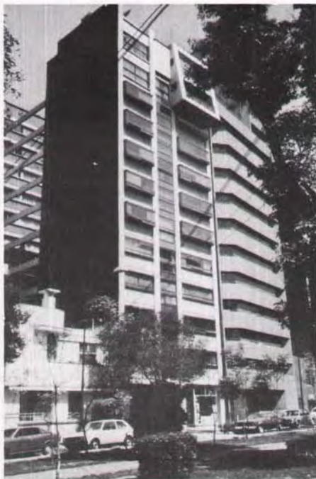
Fig. A1. Eleven-story apartment building on Amsterdam Avenue.
