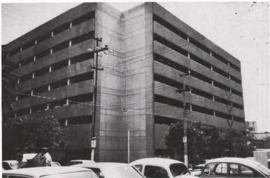
Fig. A3. Seven-story parking garage at Moreno Street.
