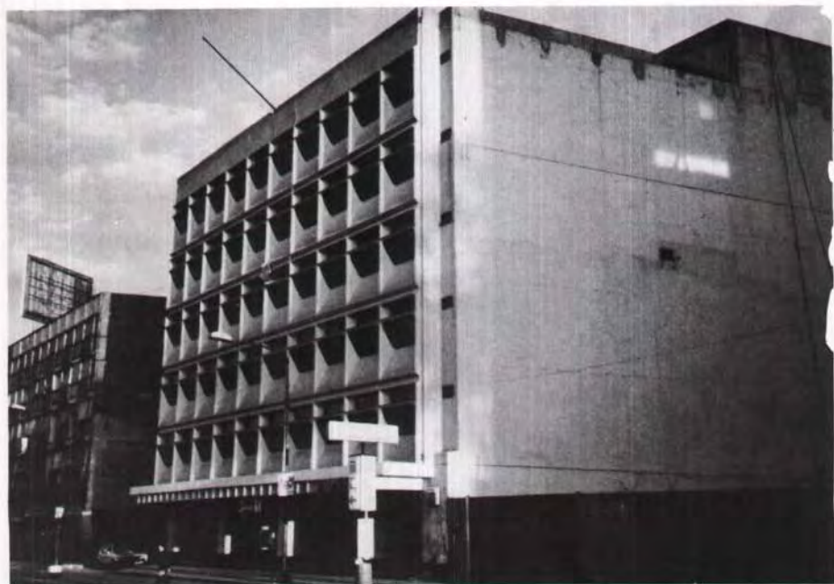
Fig. 10. Architectural precast concrete cladding.
