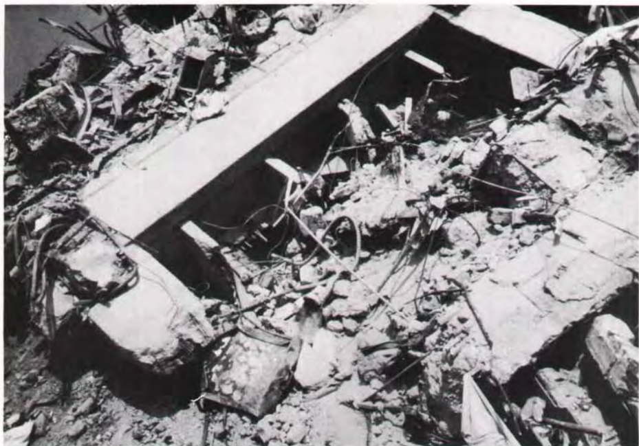
Fig. 12. Remains of six-story Maternity Ward, General Hospital.
