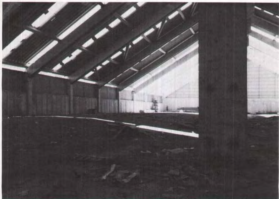
Fig. 19. Slab waves 1 m (3.3 ft) high.
