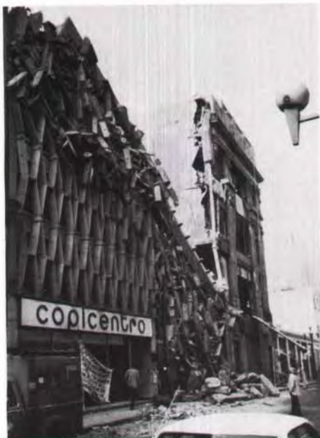
Fig. 14. Partially collapsed seven-story public parking garage at Carranza St.
