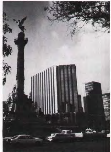
Fig. 8. Most buildings behaved well.
