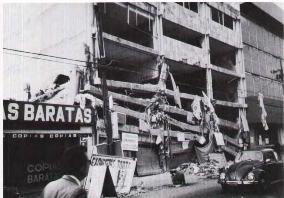
Fig. 6. Collapsed middle stories.
