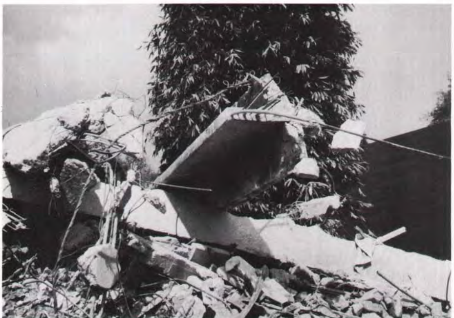
Fig. 13. Remains of six-story Maternity Ward, General Hospital.
