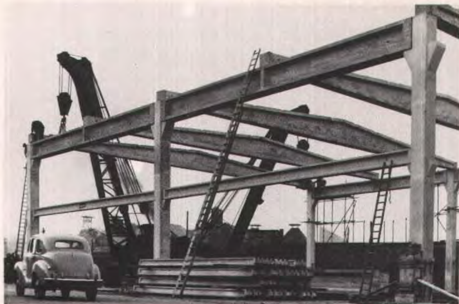
Fig. 9. Freight depot with partially prestressed concrete beams (Bury St. Edmonds, England, 1952).
