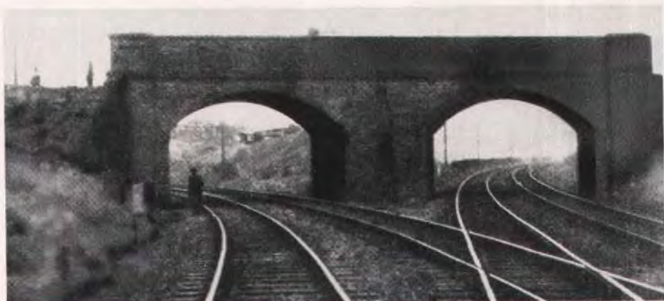
Fig. 2. Brick masonry arch bridge before reconstruction (Gorton-Manchester line).
