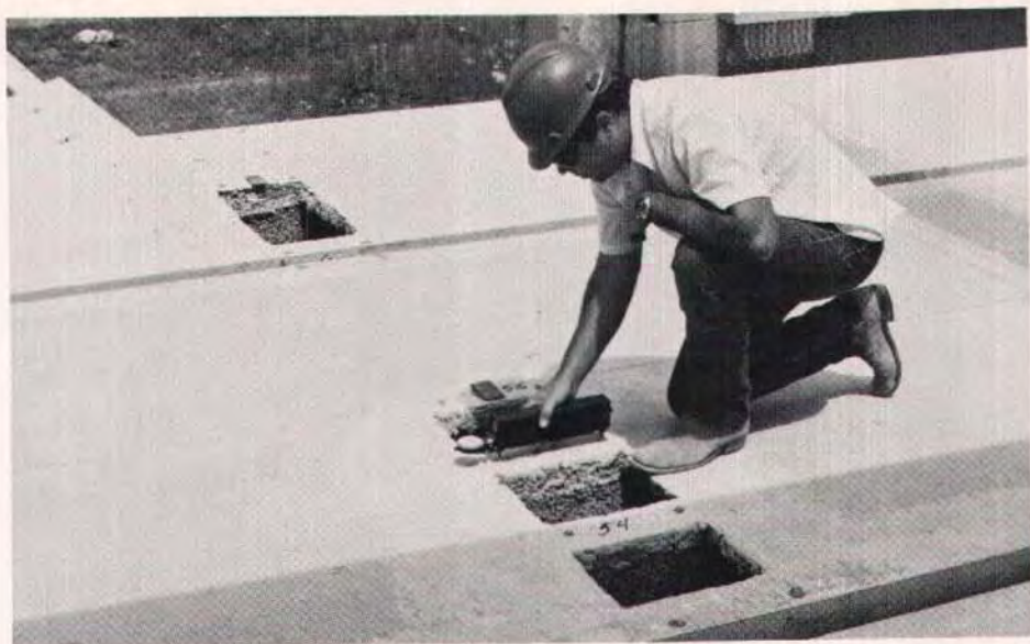
Fig. 3. Holes at midspan in Slabs 4 and 5 and Whittemore strain gage being used to measure top fiber strain.
