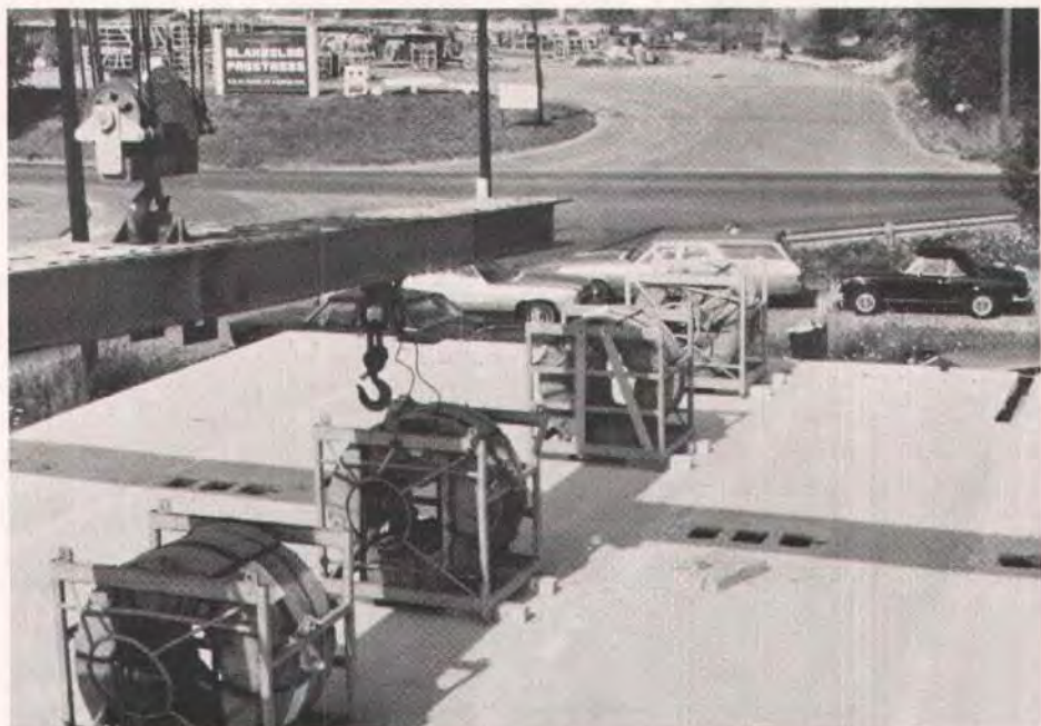
Fig. 1. Load distribution test on full-scale floor slab assembly.
