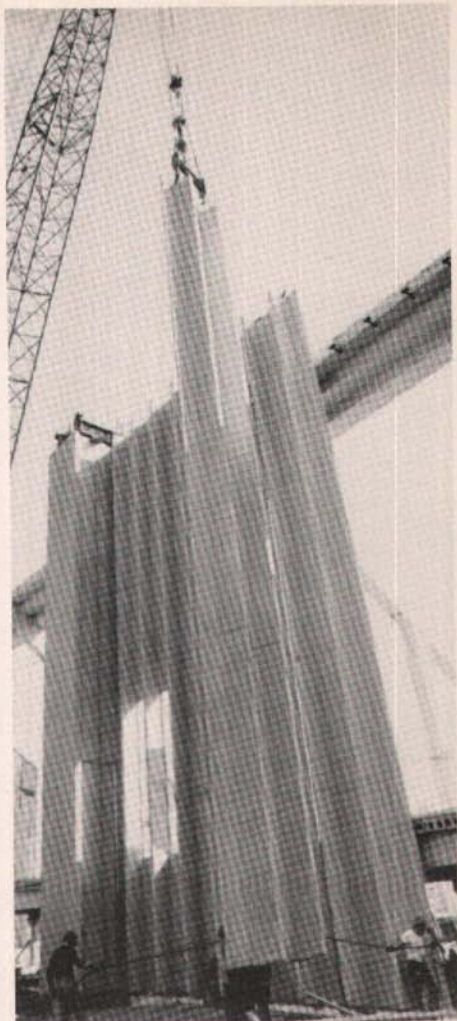
Precast twin tee column in place, adjacent column being erected.
