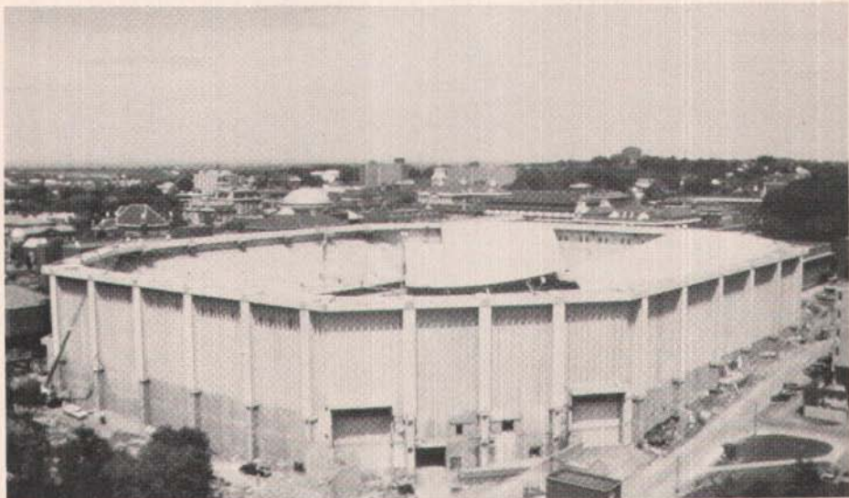
Aerial view of roof material being installed.
