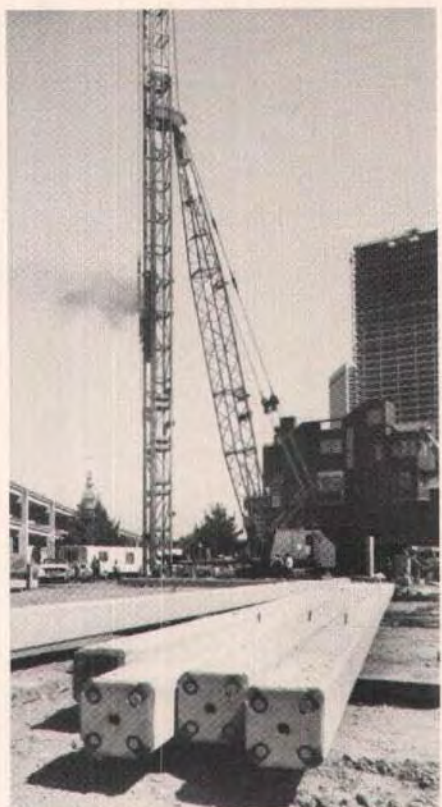
Fig. 3. Piles with wedge-type splice.
