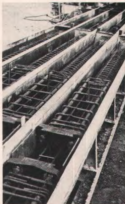
Fig. 7. Splice assembly of specimen prior to casting.
