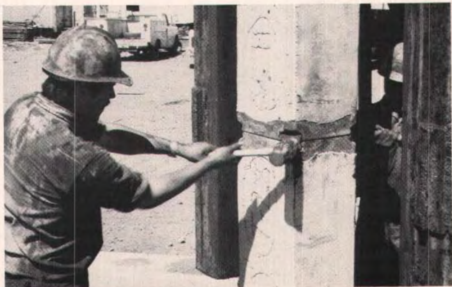
Fig. 5. Workman driving in splice wedge.
