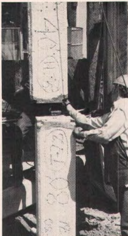
Fig. 4. Positioning of upper pile section.
