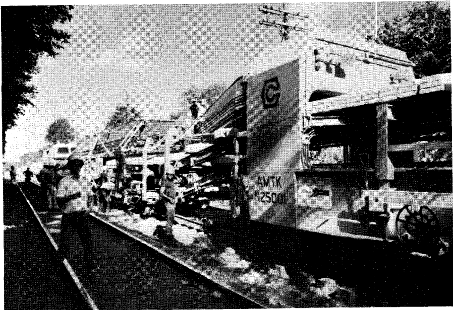
Fig. 28. Track renewal machine.
