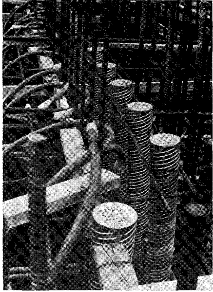
Fig. 12. Series of capped sheaths at base of Tower shaft.
