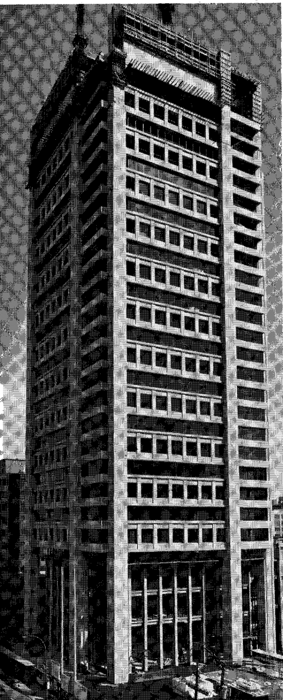
Fig. 19. ICAO Tower nearing completion (1974).
