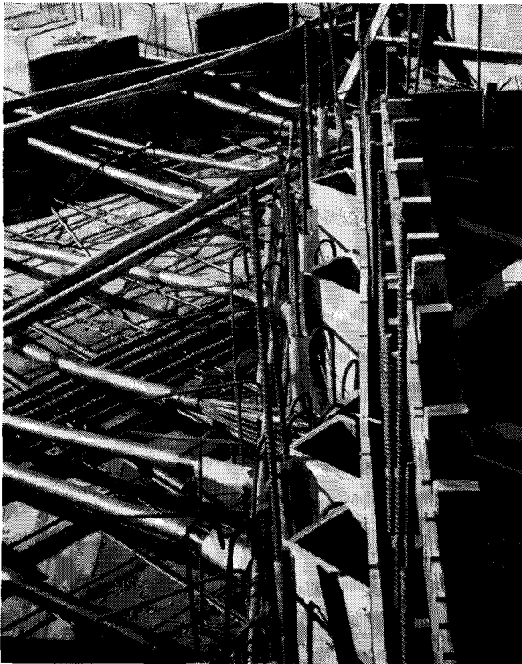
Fig. 9—Construction View Showing Congestion at Slab Edges
