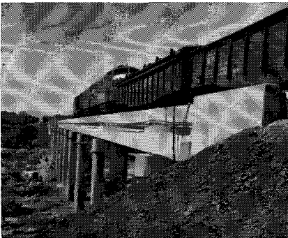
Fig. 14—Southern Pacific Co. Bridge 0.46 at Houston, Texas.
