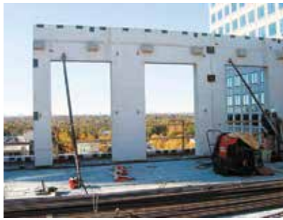
Braced precast concrete wall panel during erection.
