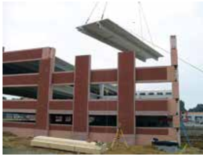
Precast Concrete double tee being installed.
